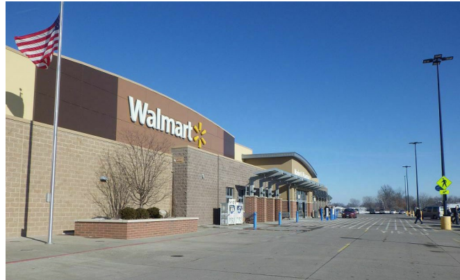
3 GRADE CONCRETE TILT-UP – STEEL FRAME
