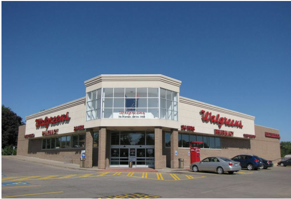
3 GRADE BRICK ON BLOCK – STEEL FRAME
