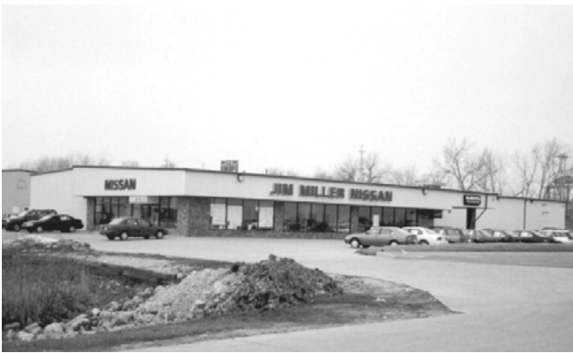
4 GRADE METAL – STEEL FRAME SERVICE AREA & BRICK ON BLOCK – STEEL FRAME SALES AREA
