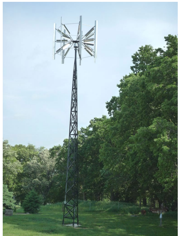
LATTICE TOWER WIND TURBINE
