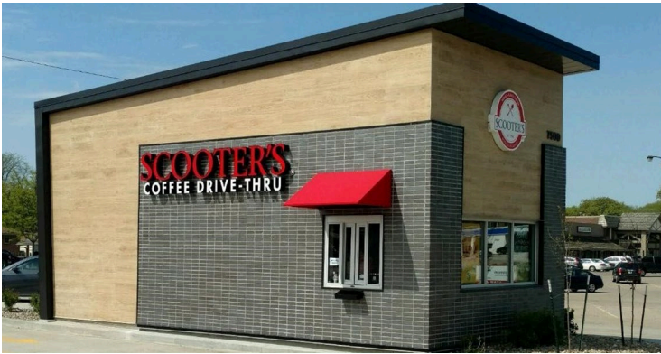
3 GRADE BRICK VENEER – WOOD FRAME
