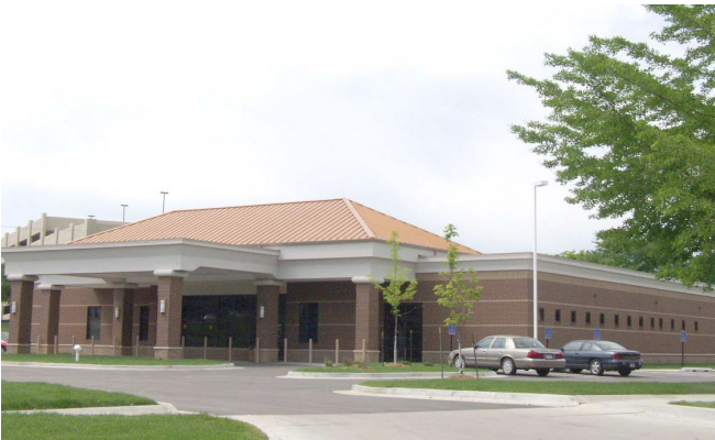
2 GRADE BRICK ON BLOCK – STEEL FRAME
