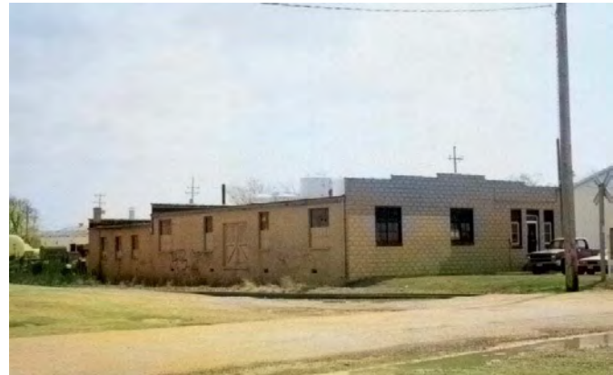
5 GRADE CONCRETE BLOCK – WOOD FRAME
