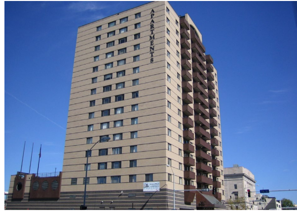
3 GRADE BRICK ON BLOCK – CONCRETE FRAME
