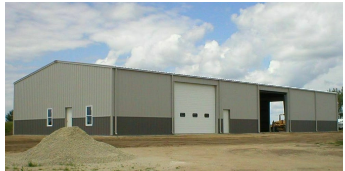
4 GRADE METAL WAREHOUSE – STEEL FRAME
