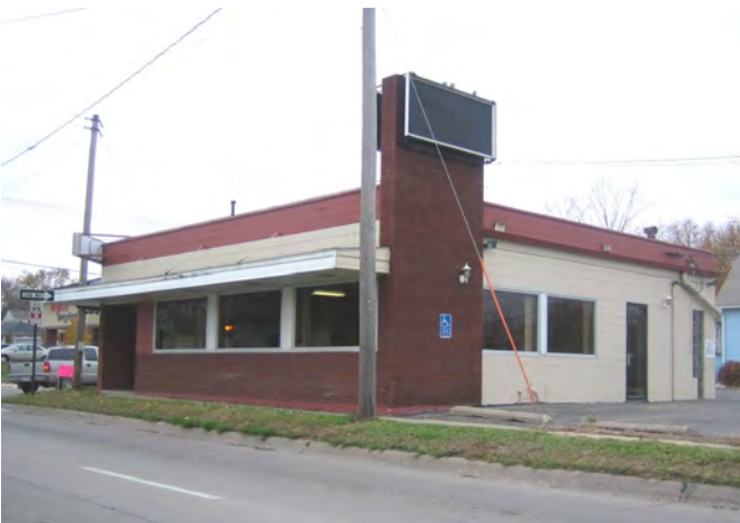
4 - 5 GRADE CONCRETE BLOCK – WOOD FRAME
