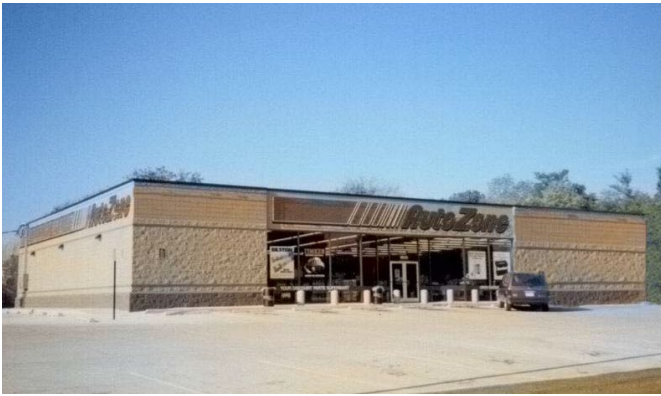
3 GRADE DECORATIVE CONCRETE BLOCK – STEEL FRAME
