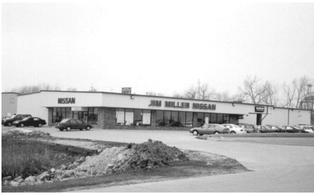
4 GRADE METAL – STEEL FRAME SERVICE AREA & BRICK ON BLOCK – STEEL FRAME SALES AREA
