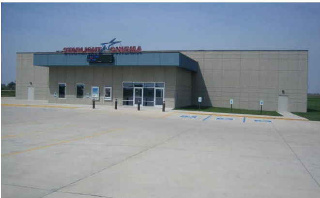
4 GRADE CONCRETE TILT-UP – STEEL FRAME
