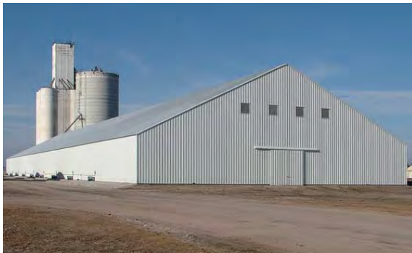
Metal – Steel Frame Flat Grain Storage
