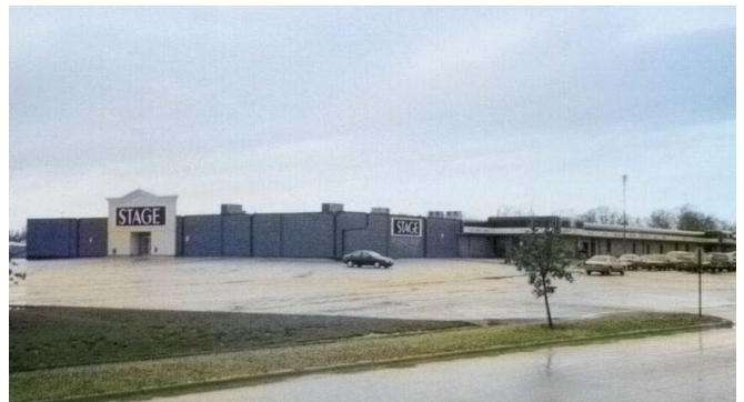
4 GRADE BRICK ON BLOCK – STEEL FRAME
