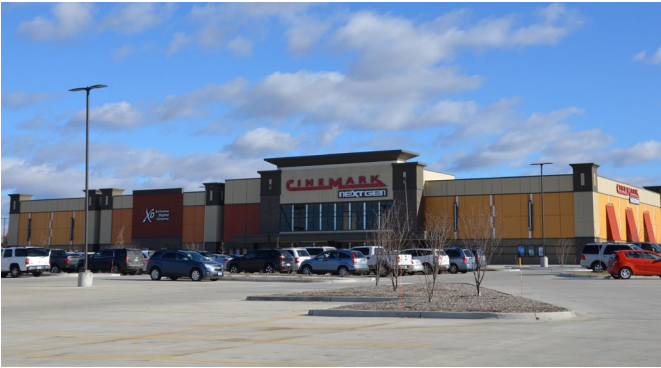
2 GRADE CONCRETE TILT-UP – STEEL FRAME
