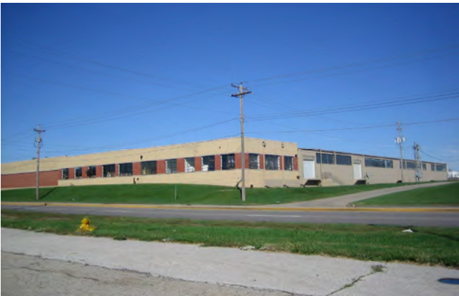
4 GRADE CONCRETE BLOCK – STEEL FRAME
