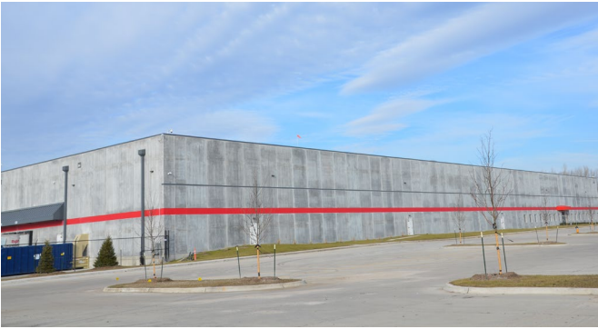
4 GRADE CONCRETE TILT-UP – STEEL FRAME
