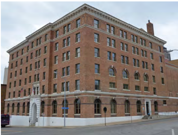
4 GRADE BRICK – STEEL FRAME
