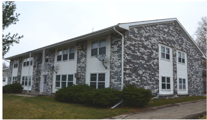
4 GRADE BRICK VENEER – WOOD FRAME
