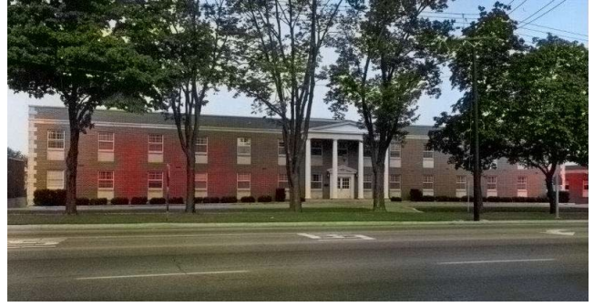
3 GRADE BRICK – REINFORCED CONCRETE FRAME
