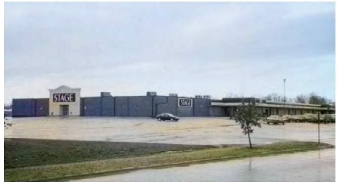
4 GRADE BRICK ON BLOCK – STEEL FRAME
