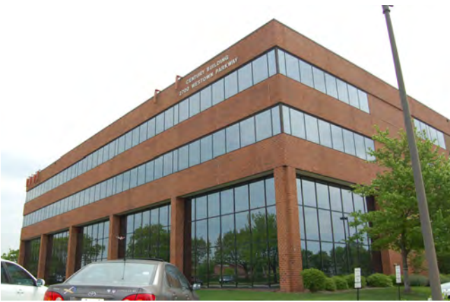
2 GRADE BRICK ON BLOCK – STEEL FRAME
