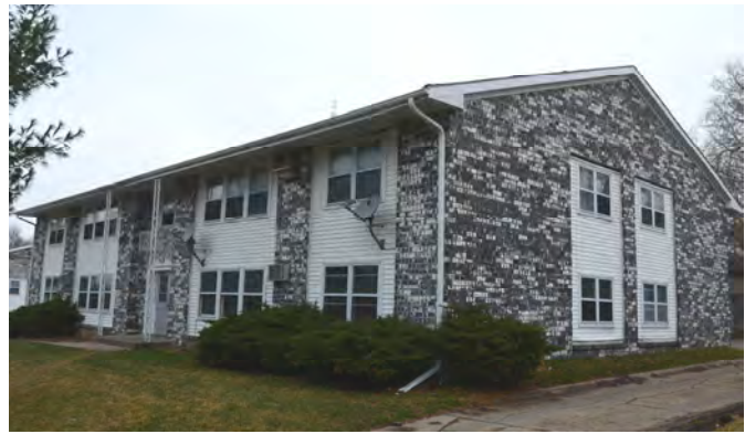
4 GRADE BRICK VENEER – WOOD FRAME
