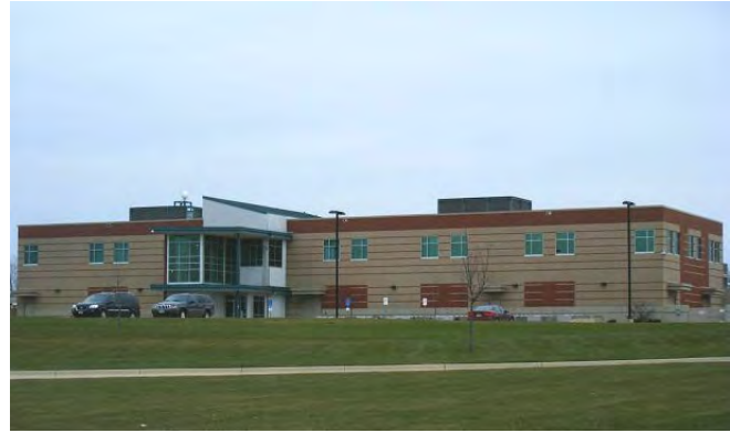
3 GRADE CONCRETE TILT-UP – STEEL FRAME
