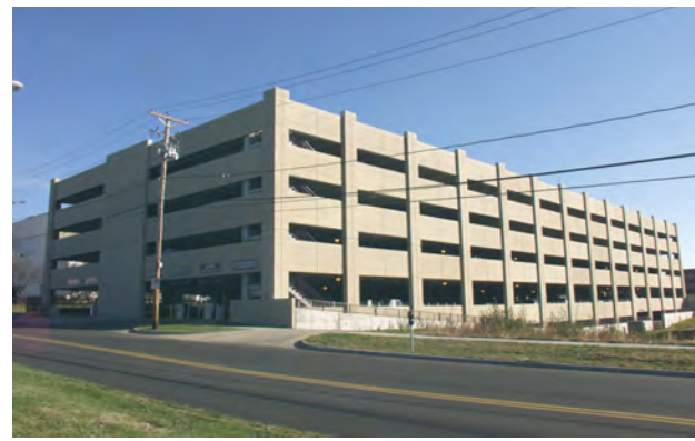
4 + 10 GRADE REINFORCED CONC. – REINFORCED CONCRETE FRAME
