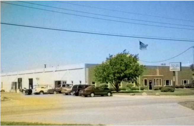
3 GRADE CONCRETE BLOCK – STEEL FRAME
