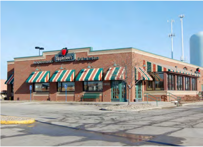
2 GRADE BRICK VENEER – STEEL FRAME
