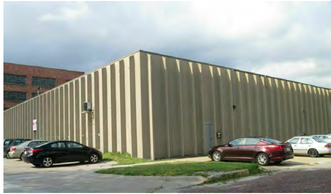
3 GRADE CONCRETE TILT-UP – CONCRETE FRAME
