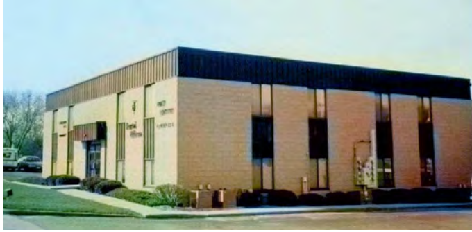
4 GRADE CONCRETE BLOCK – WOOD FRAME
