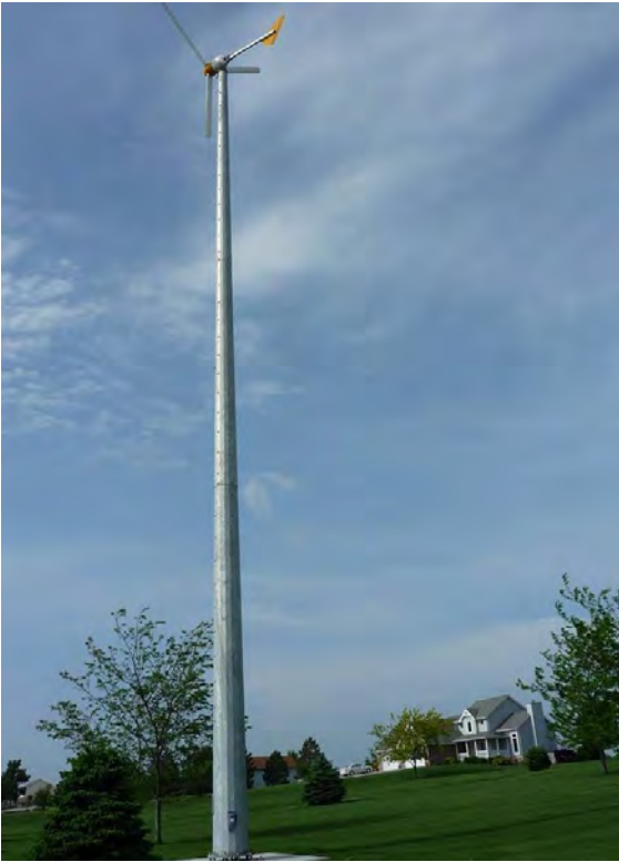
MONOPOLE TOWER WIND TURBINE
