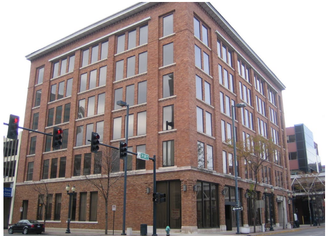
4 GRADE BRICK ON BLOCK – REINFORCED CONCRETE FRAME
