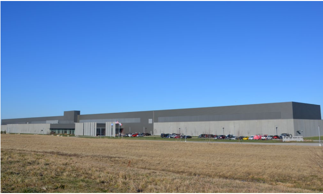
3 + 10 GRADE CONCRETE TILT-UP – STEEL FRAME
