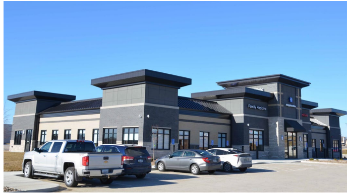
2 GRADE BRICK VENEER – WOOD FRAME
