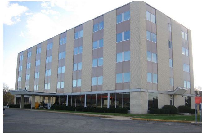
4 GRADE BRICK ON BLOCK – REINFORCED CONCRETE FRAME
