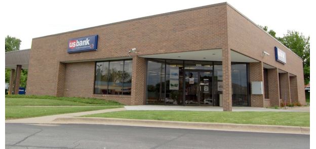
3 GRADE BRICK - STEEL FRAME
