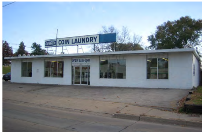
5 GRADE CONCRETE BLOCK – WOOD FRAME
