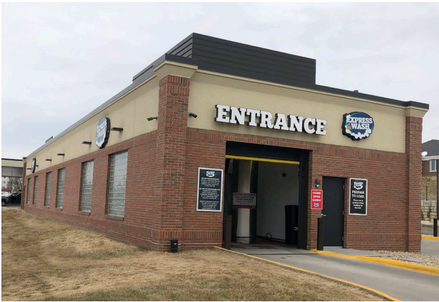
2 GRADE – DRIVE THRU BRICK – STEEL FRAME
