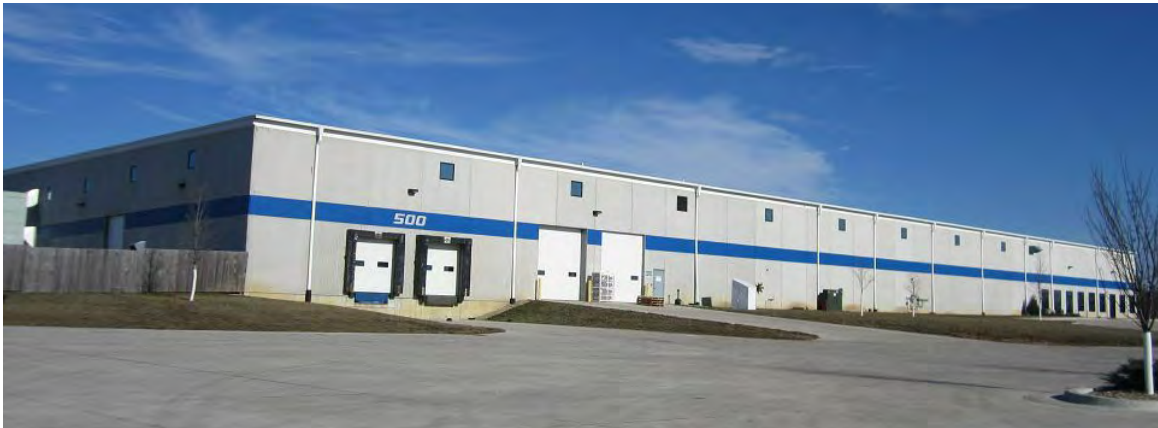
4 GRADE CONCRETE TILT-UP – STEEL FRAME
