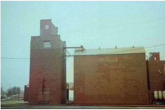
CRIBBED ELEVATOR WITH CRIBBED ANNEX
