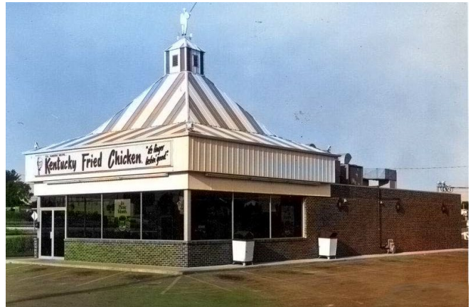
4 GRADE BRICK ON BLOCK – STEEL FRAME
