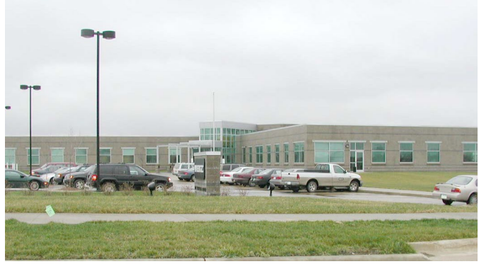
2 GRADE BRICK – STEEL FRAME
