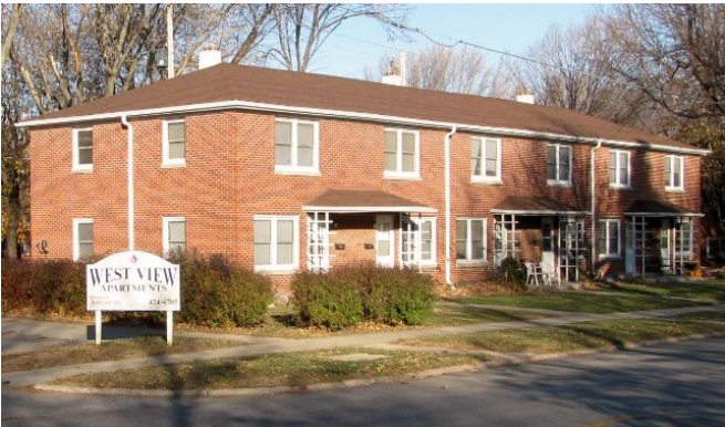
4 GRADE BRICK VENEER – WOOD FRAME
