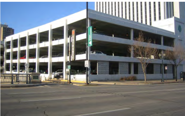
4 GRADE REINFORCED CONC. – REINFORCED CONCRETE FRAME
