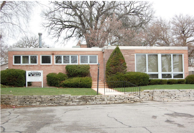
4 GRADE BRICK ON BLOCK – STEEL FRAME
