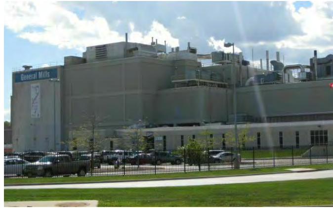
3 GRADE CONCRETE TILT-UP – STEEL FRAME
