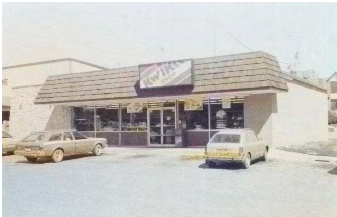
5 GRADE CONCRETE BLOCK – STEEL FRAME
