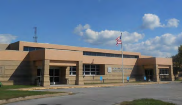
2 GRADE BRICK ON BLOCK – STEEL FRAME
