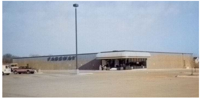
4 GRADE CONCRETE TILT-UP – STEEL FRAME
