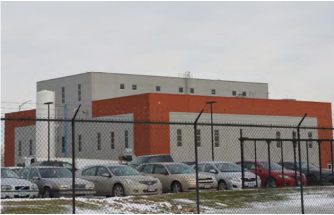
2 GRADE CONCRETE TILT-UP – CONCRETE FRAME
