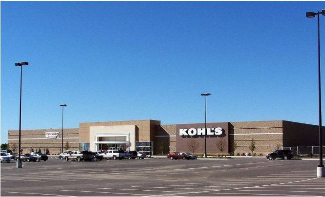
3 GRADE BRICK ON BLOCK – STEEL FRAME
