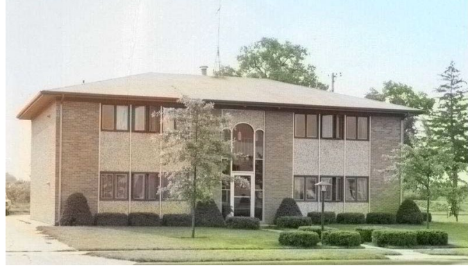
4 + 10 GRADE BRICK VENEER – WOOD FRAME
