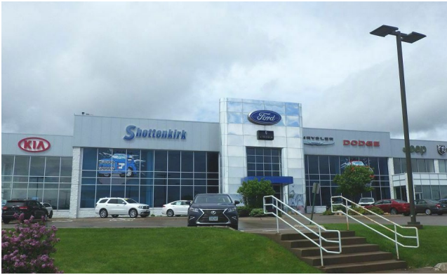
2 GRADE DECORATIVE CONCRETE BLOCK – STEEL FRAME
