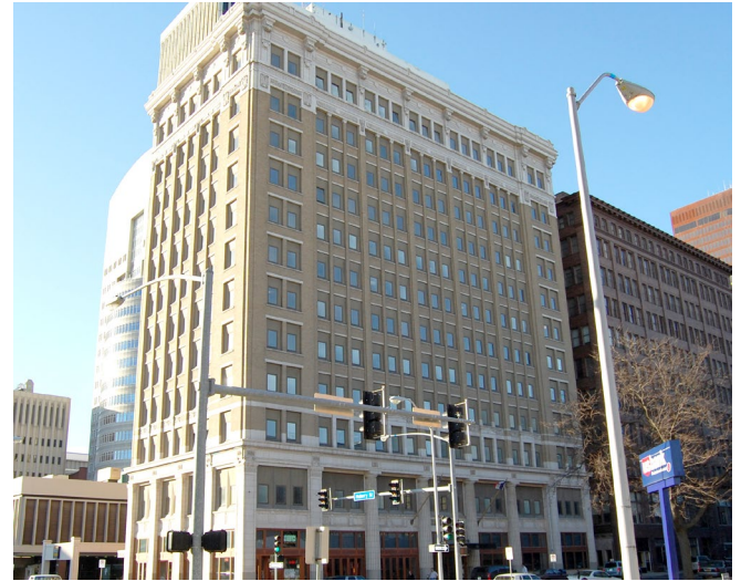
3 GRADE BRICK ON BLOCK – STEEL FRAME
