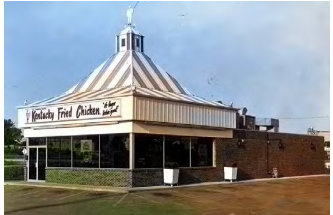
4 GRADE BRICK ON BLOCK – STEEL FRAME
