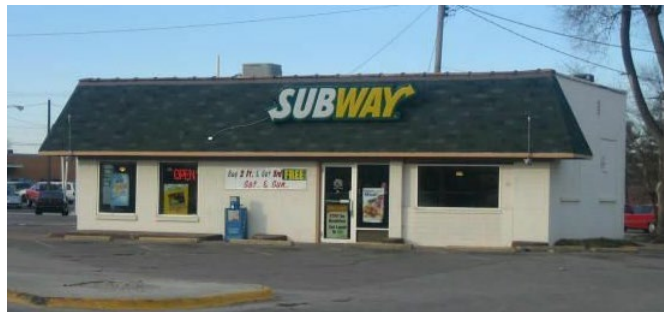
5 GRADE BRICK ON CONCRETE BLOCK – WOOD FRAME
