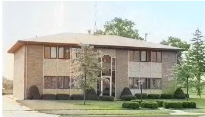
4 + 10 GRADE BRICK VENEER – WOOD FRAME
