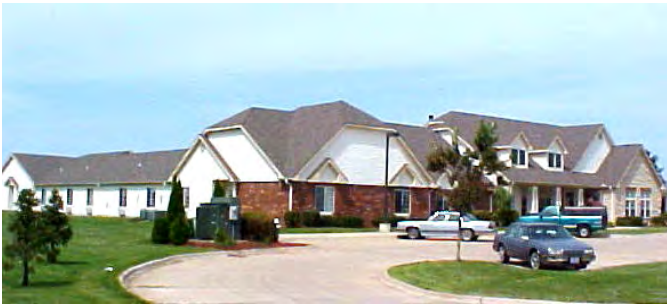
3 + 10 GRADE BRICK VENEER – WOOD FRAME
