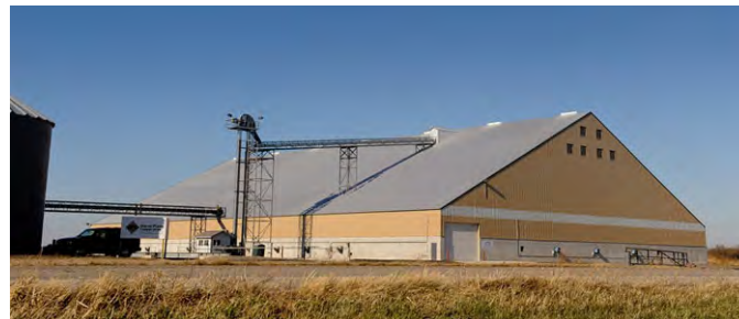
Reinforced Concrete w/ Metal – Steel Frame above Flat Grain Storage
