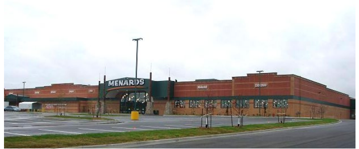
3 GRADE CONCRETE TILT-UP – STEEL FRAME
