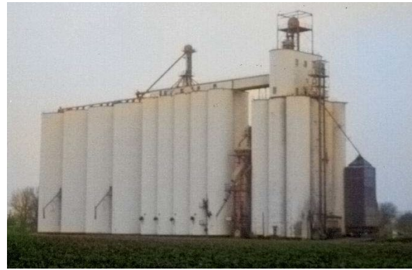
CONCRETE ELEVATOR WITH CONCRETE ANNEX
