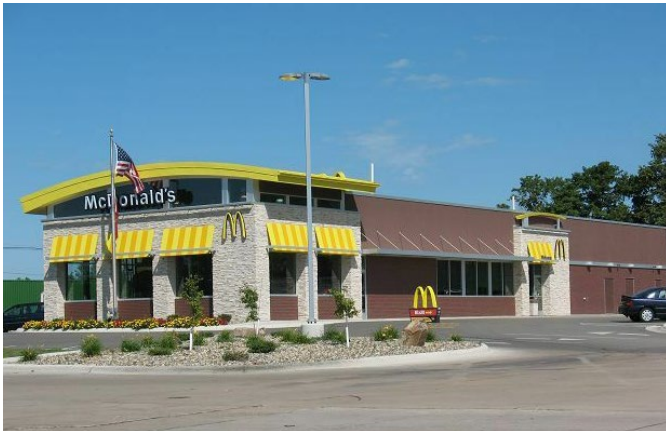
2 GRADE BRICK VENEER – WOOD FRAME
