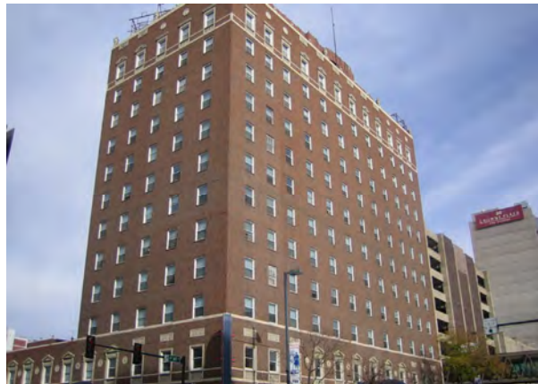
4 GRADE BRICK ON BLOCK – CONCRETE FRAME
