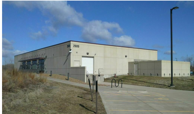
4 GRADE CONCRETE TILT-UP – STEEL FRAME
