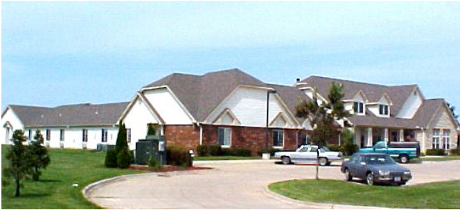
3 + 10 GRADE BRICK VENEER – WOOD FRAME
