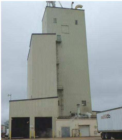
4 GRADE METAL FEED MILL W/ DISTRIBUTION FLOOR
