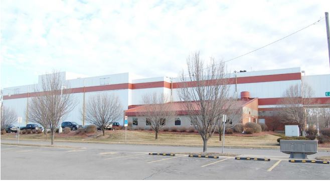
3 GRADE PRE-ENGINEERED SANDWICH PANEL – STEEL FRAME
