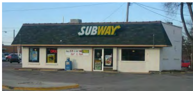
5 GRADE BRICK ON CONCRETE BLOCK – WOOD FRAME
