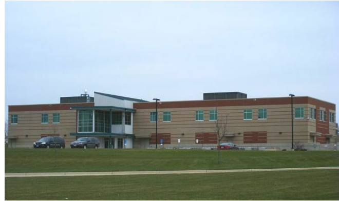
3 GRADE CONCRETE TILT-UP – STEEL FRAME
