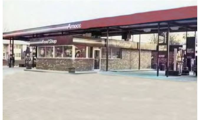
4 GRADE BRICK ON BLOCK – STEEL FRAME
