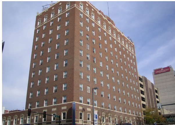
4 GRADE BRICK ON BLOCK – CONCRETE FRAME
