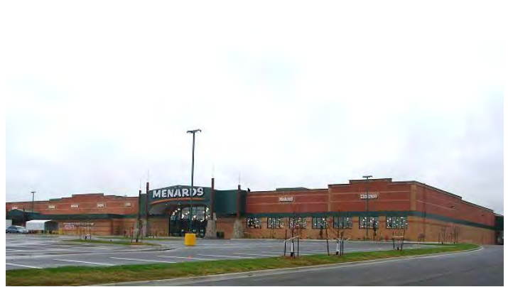
3 GRADE CONCRETE TILT-UP – STEEL FRAME
