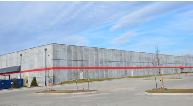
4 GRADE CONCRETE TILT-UP – STEEL FRAME
