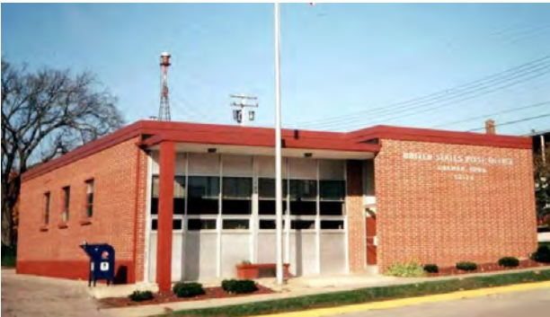
4 GRADE BRICK ON BLOCK – STEEL FRAME
