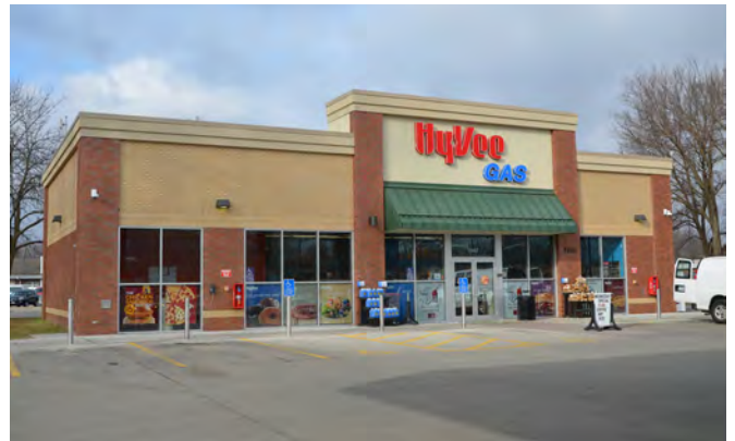
2 GRADE BRICK VENEER – STEEL FRAME
