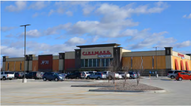
2 GRADE CONCRETE TILT-UP – STEEL FRAME
