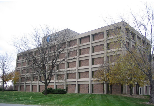
3 GRADE BRICK ON BLOCK – REINFORCED CONCRETE FRAME
