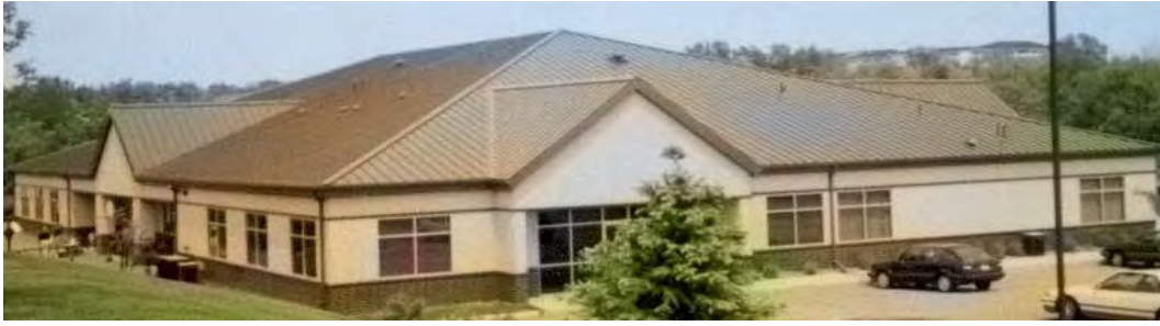
3 GRADE CONCRETE BLOCK – WOOD FRAME
