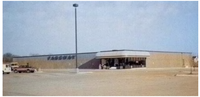
4 GRADE CONCRETE TILT-UP – STEEL FRAME
