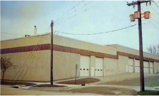
3 GRADE CONCRETE BLOCK – WOOD FRAME
