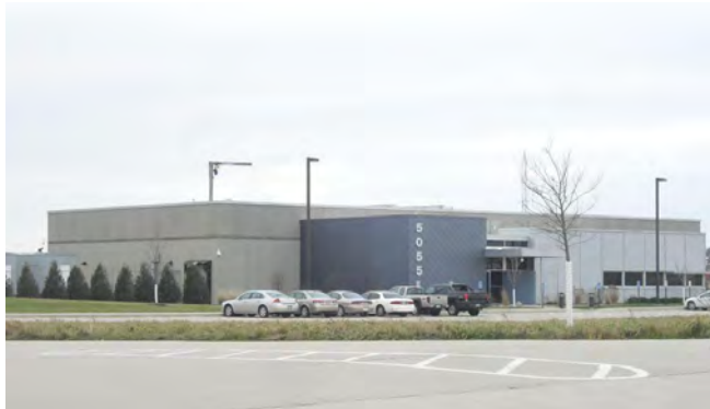
4 GRADE CONCRETE TILT-UP – STEEL FRAME
