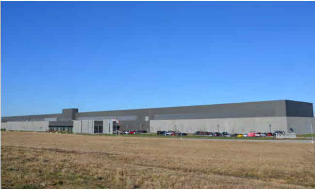
3 + 10 GRADE CONCRETE TILT-UP – STEEL FRAME
