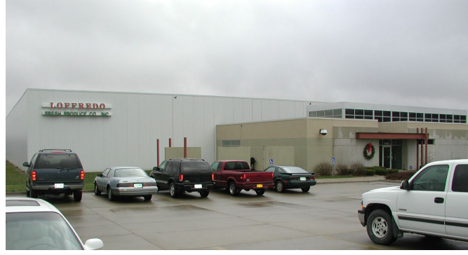
4 GRADE PRE-ENGINEERED SANDWICH PANEL – STEEL FRAME
