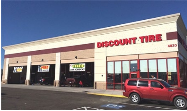
2 GRADE DECORATIVE CONCRETE BLOCK – STEEL FRAME
