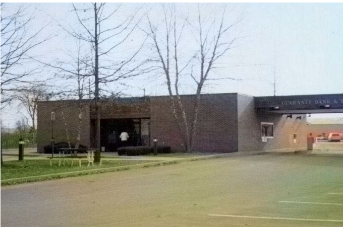
4 GRADE BRICK – STEEL FRAME
