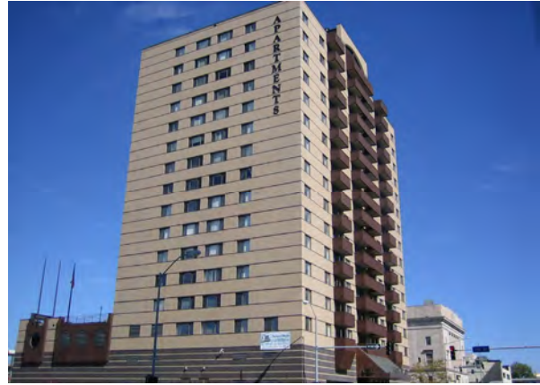
3 GRADE BRICK ON BLOCK – CONCRETE FRAME
