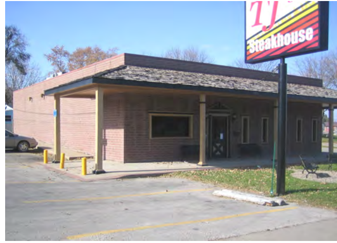
4 GRADE BRICK ON BLOCK – WOOD FRAME
