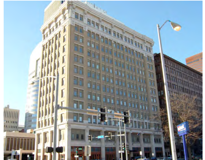
3 GRADE BRICK ON BLOCK – STEEL FRAME
