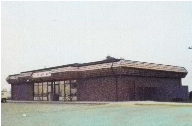
3 GRADE BRICK ON CONCRETE BLOCK – WOOD FRAME
