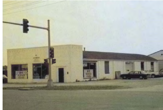
5 GRADE CONCRETE BLOCK – WOOD FRAME
