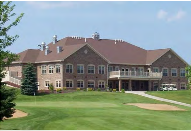
2 GRADE BRICK VENEER – WOOD FRAME
