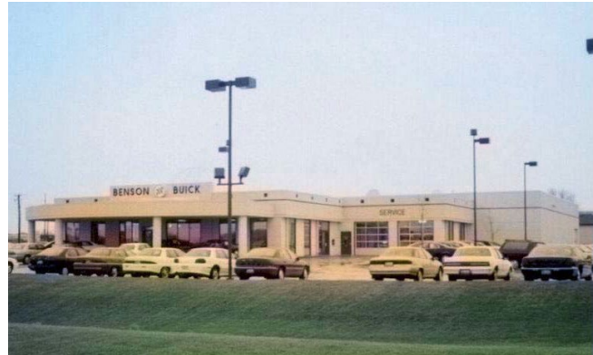
3 + 10 GRADE EIFS ON MASONRY – STEEL FRAME
