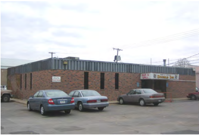
4 GRADE BRICK ON BLOCK – STEEL FRAME
