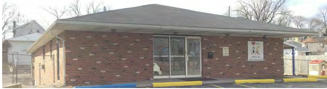
4 GRADE BRICK VENEER – WOOD FRAME
