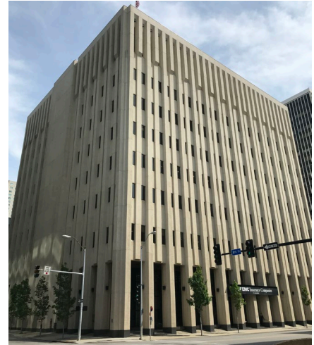
2 GRADE CONCRETE – STEEL FRAME
