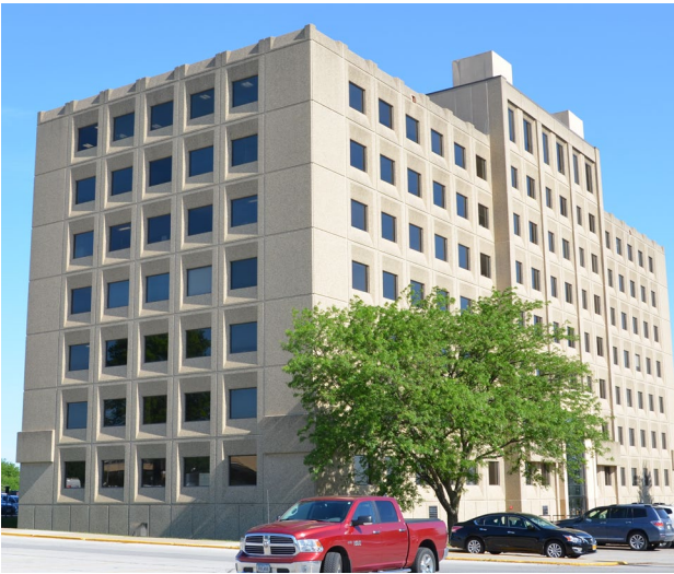
3 GRADE CONCRETE – CONCRETE FRAME
