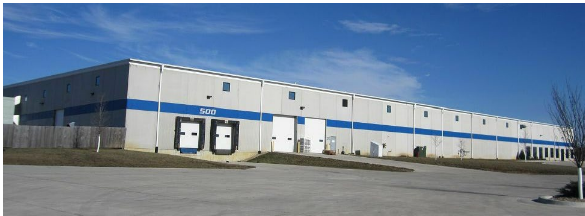
4 GRADE CONCRETE TILT-UP – STEEL FRAME
