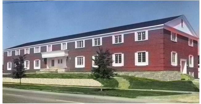
4 + 5 GRADE BRICK VENEER – WOOD FRAME
