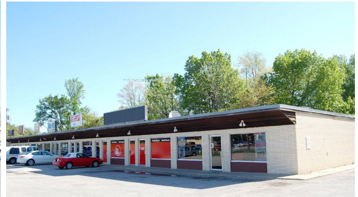
4 – 10 GRADE BRICK – STEEL FRAME
