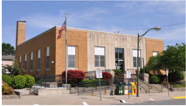
3 GRADE BRICK ON BLOCK – STEEL FRAME
