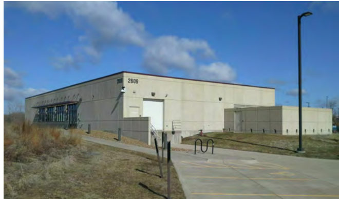
4 GRADE CONCRETE TILT-UP – STEEL FRAME
