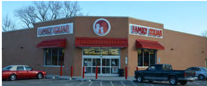
3 GRADE BRICK VENEER – STEEL FRAME
