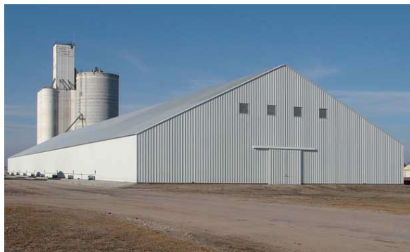
Metal – Steel Frame Flat Grain Storage
