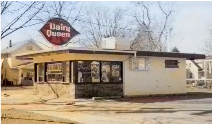
5 GRADE CONCRETE BLOCK – WOOD FRAME
