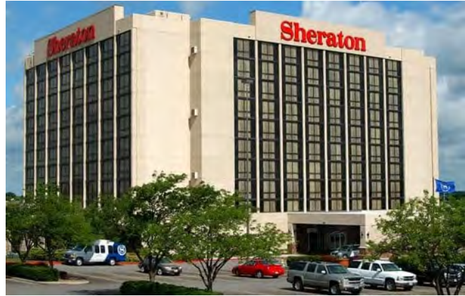
2 GRADE CONCRETE TILT-UP – STEEL FRAME
