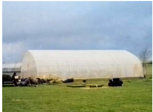
4 GRADE POLYETHYLENE "HOOP HOUSE"
