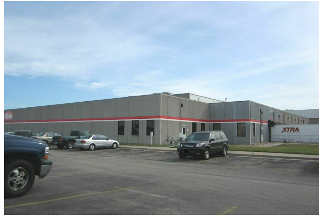
4 + 10 GRADE CONCRETE TILT-UP – STEEL FRAME
