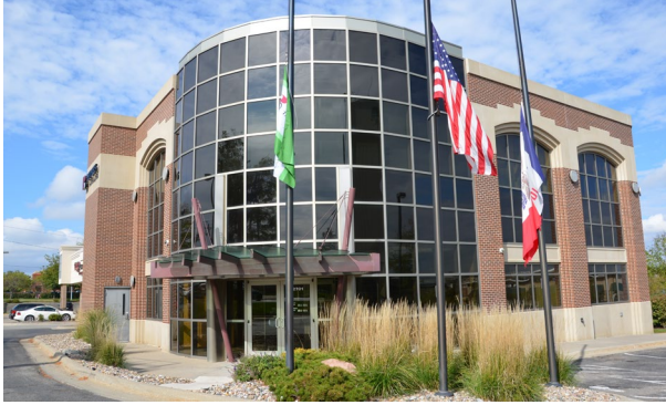
1 GRADE BRICK – STEEL FRAME
