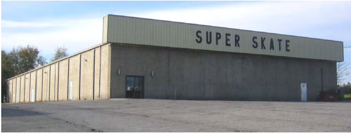
4 GRADE CONCRETE BLOCK – STEEL FRAME
