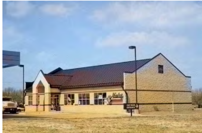
2 GRADE DECORATIVE CONCRETE BLOCK – WOOD FRAME
