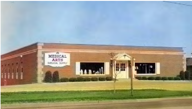
3 + 5 GRADE BRICK – REINFORCED CONCRETE FRAME
