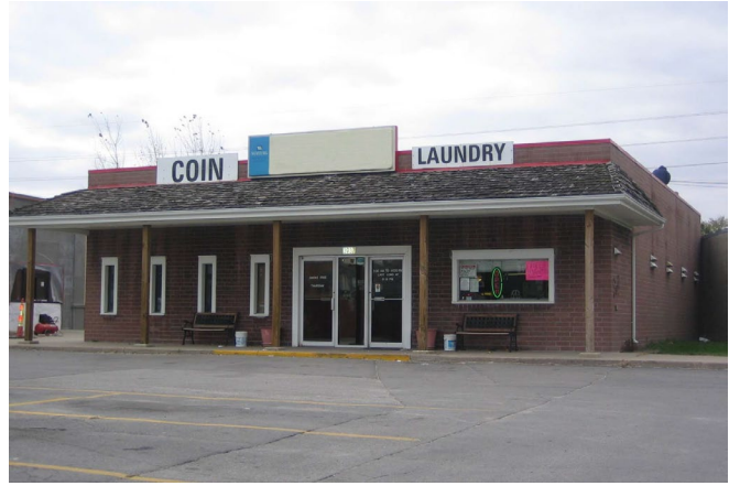
4 GRADE BRICK ON BLOCK – STEEL FRAME
