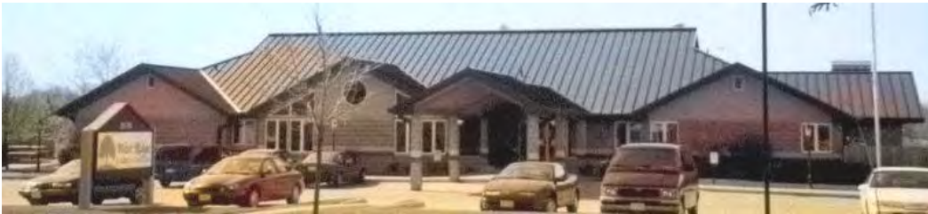
3 GRADE CONCRETE BLOCK – WOOD FRAME
