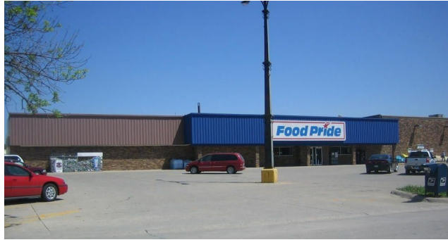
4 GRADE METAL – STEEL FRAME (BRICK STORE FRONT)
