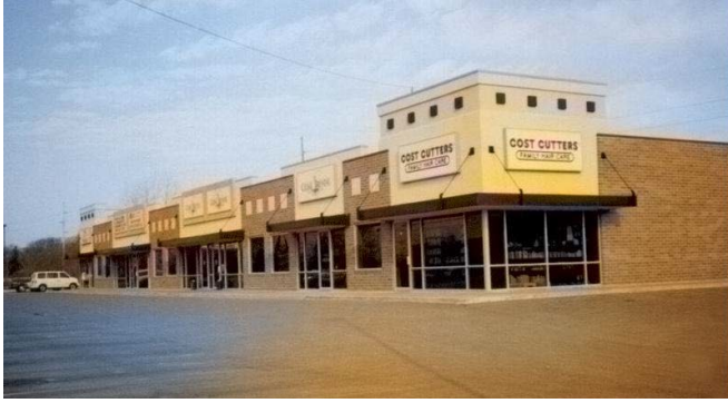
3 GRADE BRICK – STEEL FRAME
