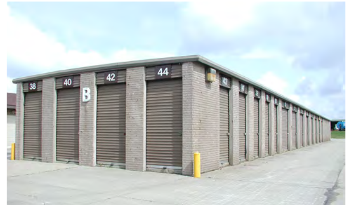
4 GRADE CONCRETE – STEEL FRAME
