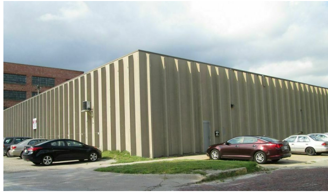
3 GRADE CONCRETE TILT-UP – CONCRETE FRAME
