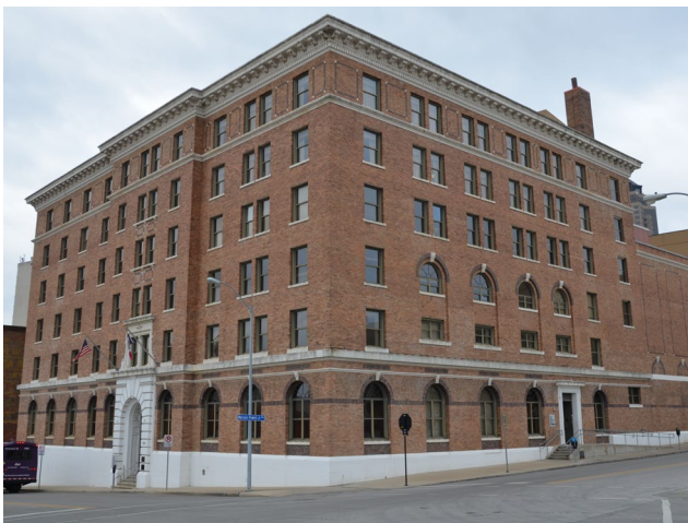
4 GRADE BRICK – STEEL FRAME
