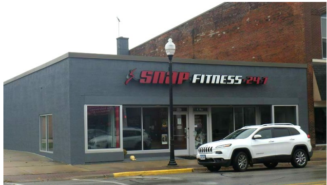
4 GRADE BRICK ON BLOCK – STEEL FRAME
