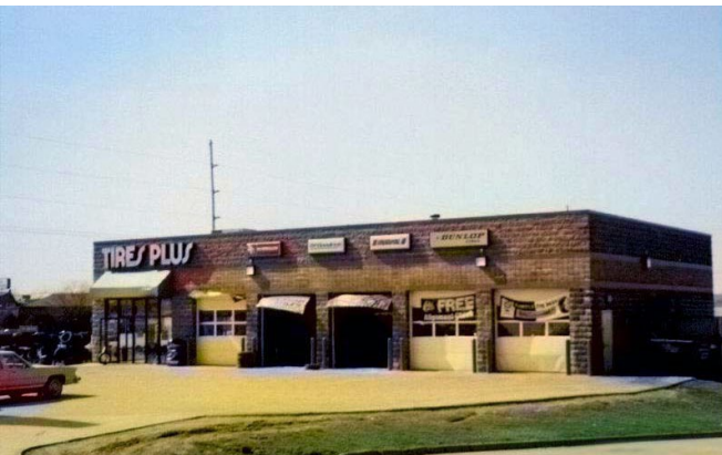
4 + 5 GRADE DECORATIVE CONCRETE BLOCK – STEEL FRAME
