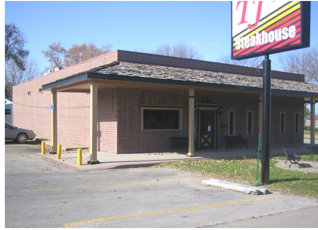
4 GRADE BRICK ON BLOCK – WOOD FRAME
