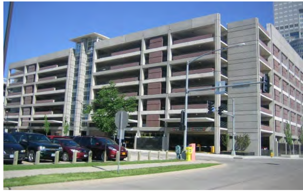
3 GRADE REINFORCED CONC. – REINFORCED CONCRETE FRAME
