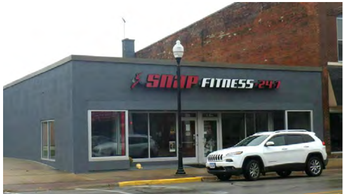
4 GRADE BRICK ON BLOCK – STEEL FRAME
