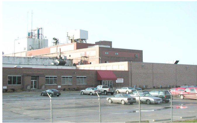
4 GRADE BRICK – STEEL FRAME
