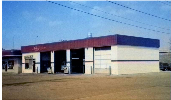
4 GRADE DECORATIVE CONCRETE BLOCK – STEEL FRAME
