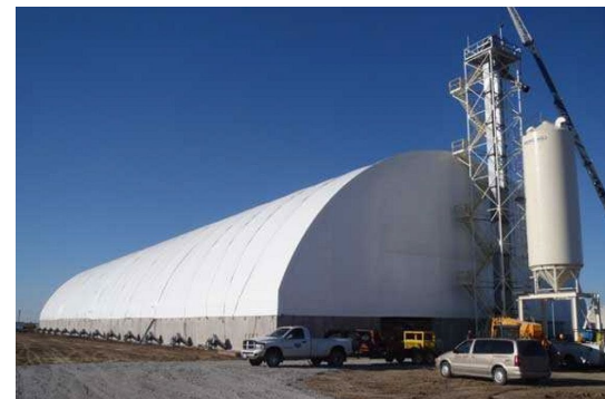
Concrete w/ Hoop Structure Flat Grain Storage
