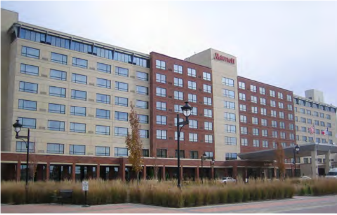
1 GRADE BRICK & REINFORCED CONCRETE – STEEL FRAME
