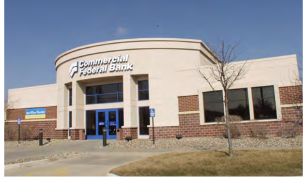
2 GRADE BRICK VENEER – STEEL FRAME
