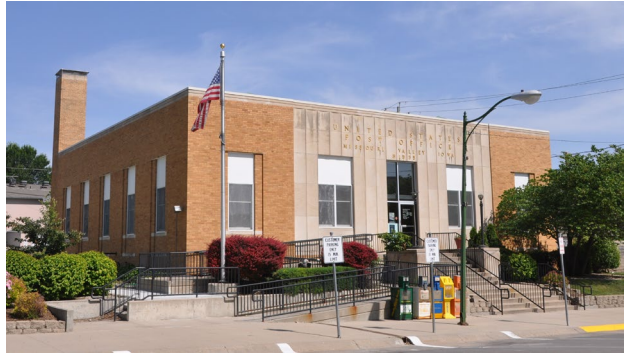
3 GRADE BRICK ON BLOCK – STEEL FRAME
