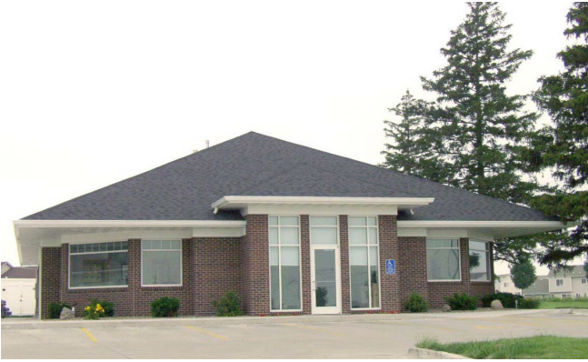
3 GRADE BRICK VENEER – WOOD FRAME
