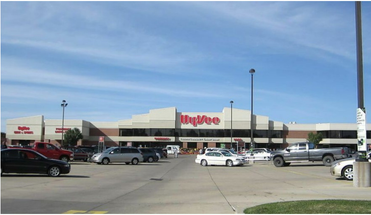
2 GRADE CONCRETE TILT-UP – STEEL FRAME
