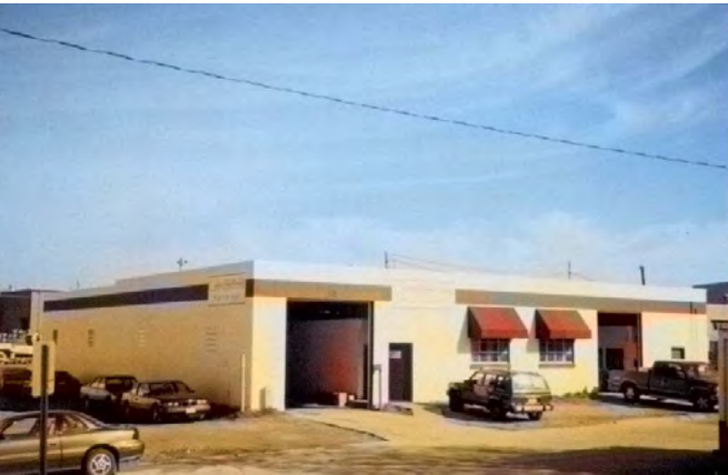
4 GRADE CONCRETE BLOCK – STEEL FRAME
