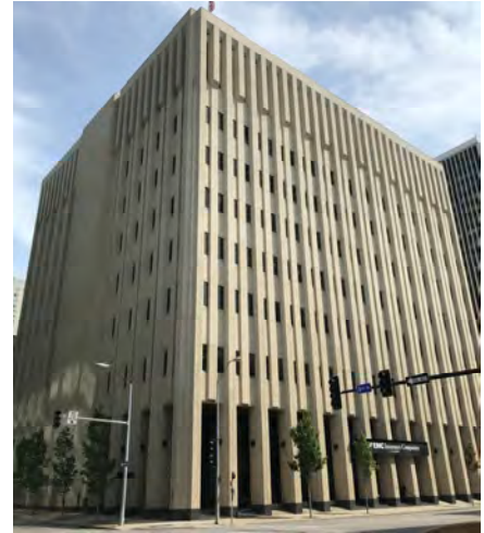
2 GRADE CONCRETE – STEEL FRAME
