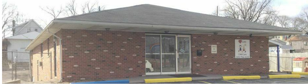
4 GRADE BRICK VENEER – WOOD FRAME
