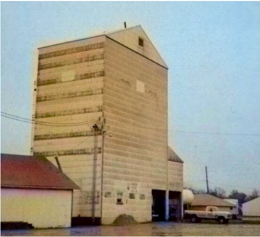
4 GRADE CRIBBED FEED MILL W/ DISTRIBUTION FLOOR
