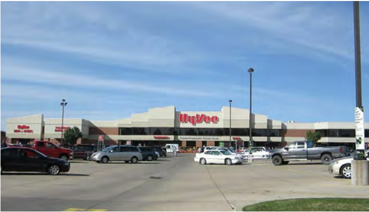
2 GRADE CONCRETE TILT-UP – STEEL FRAME
