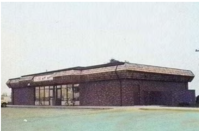
3 GRADE BRICK ON CONCRETE BLOCK – WOOD FRAME
