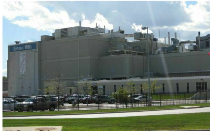
3 GRADE CONCRETE TILT-UP – STEEL FRAME
