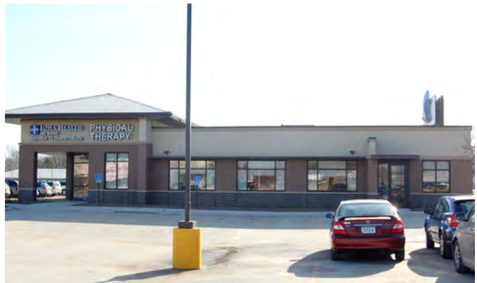
3 GRADE BRICK VENEER – STEEL FRAME
