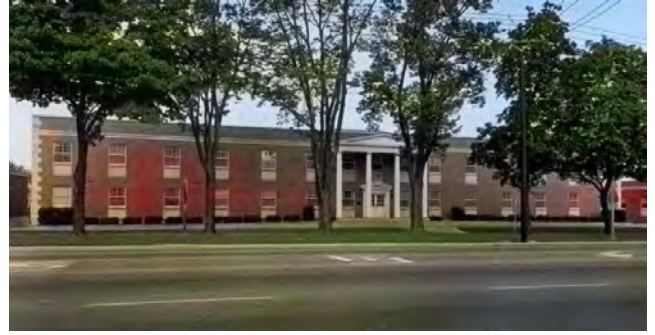
3 GRADE BRICK – REINFORCED CONCRETE FRAME
