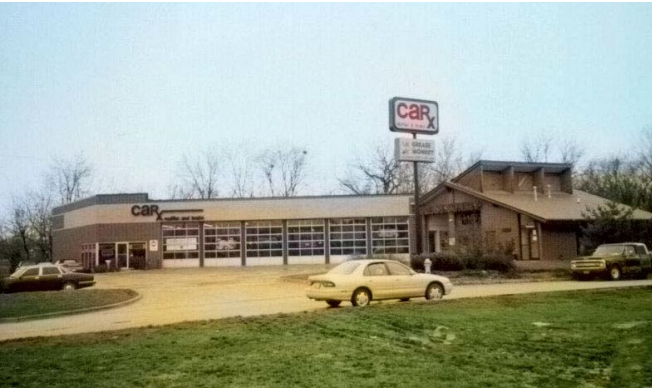
3 GRADE BRICK ON BLOCK – STEEL FRAME
