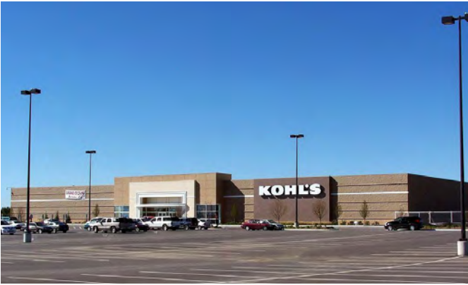
3 GRADE BRICK ON BLOCK – STEEL FRAME
