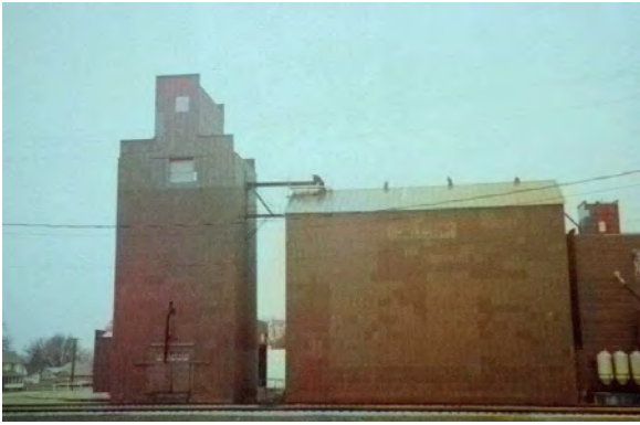
CRIBBED ELEVATOR WITH CRIBBED ANNEX
