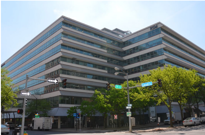
1 GRADE CONCRETE – CONCRETE FRAME
