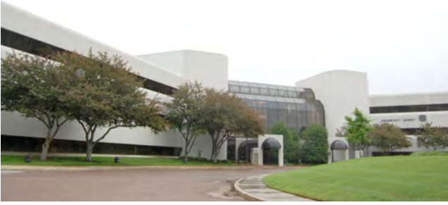
1 GRADE CONCRETE – STEEL FRAME
