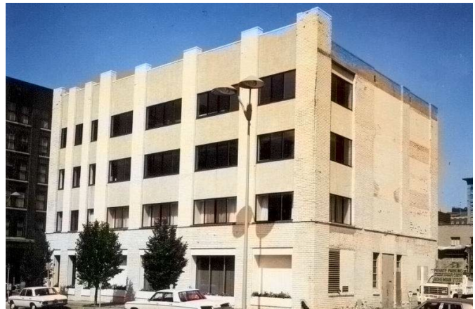
5 + 5 GRADE SOLID BRICK – STEEL FRAME
