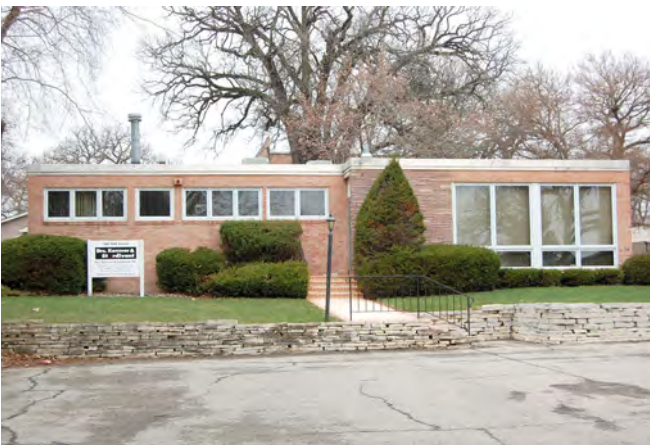
4 GRADE BRICK ON BLOCK – STEEL FRAME
