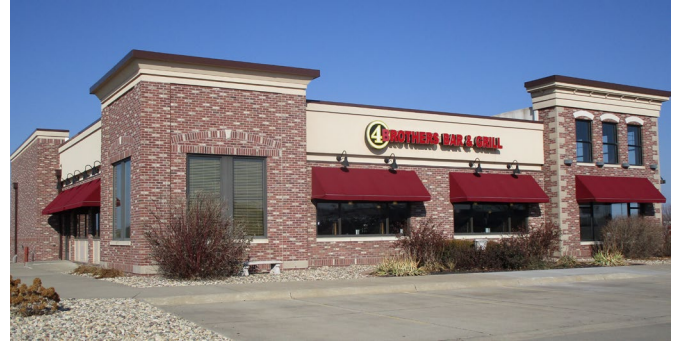
2 GRADE BRICK VENEER – WOOD FRAME
