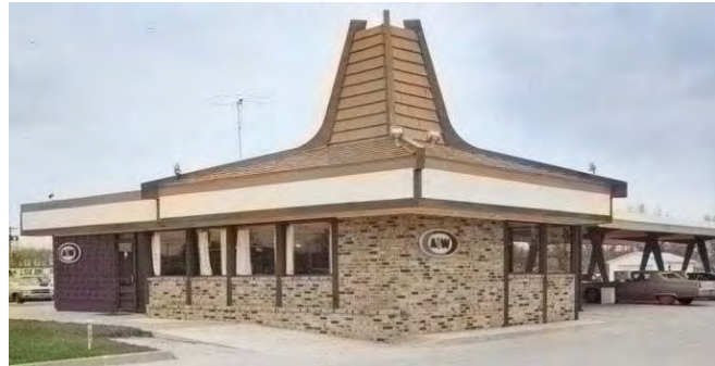
3 GRADE BRICK VENEER – STEEL FRAME
