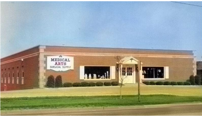
3 + 5 GRADE BRICK – REINFORCED CONCRETE FRAME
