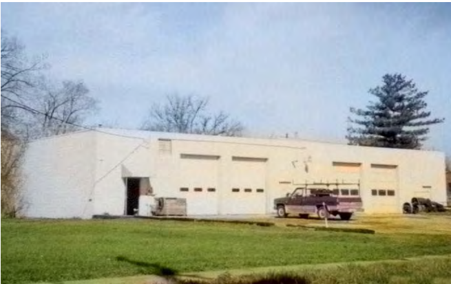
4 GRADE CONCRETE BLOCK – STEEL FRAME
