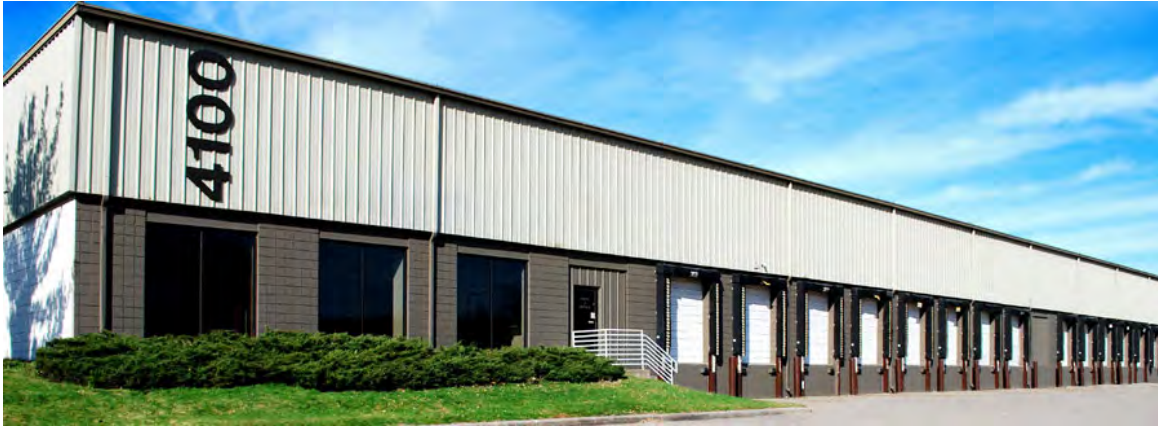
4 GRADE CONCRETE BLOCK – STEEL FRAME
