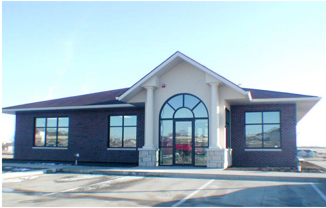
3 + 10 GRADE BRICK VENEER – WOOD FRAME
