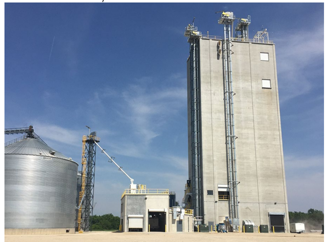
3 GRADE REINFORCED CONCRETE FEED MILL W/ DISTRIBUTION FLOOR
