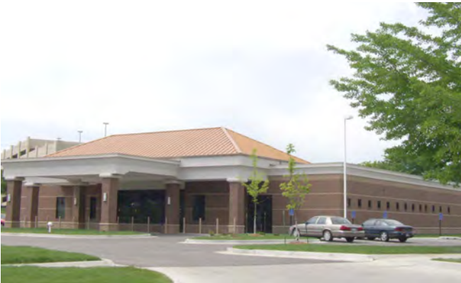
2 GRADE BRICK ON BLOCK – STEEL FRAME
