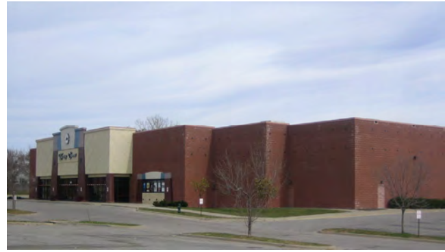
3 GRADE DECORATED CONCRETE BLOCK – STEEL FRAME
