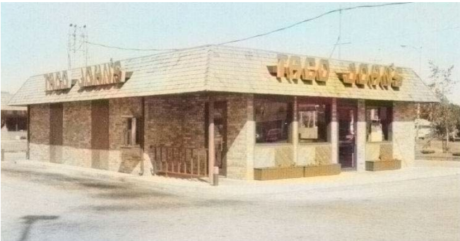
3 GRADE BRICK VENEER – WOOD FRAME
