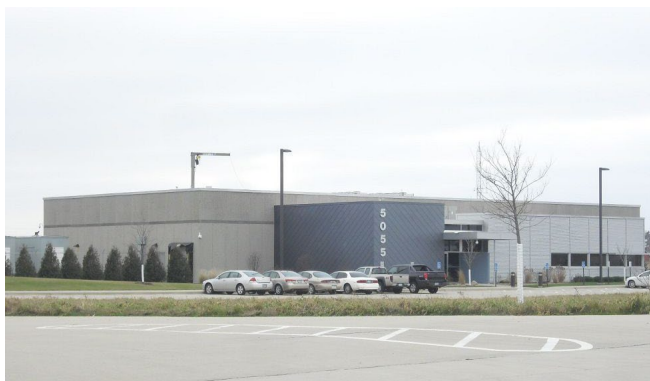
4 GRADE CONCRETE TILT-UP – STEEL FRAME
