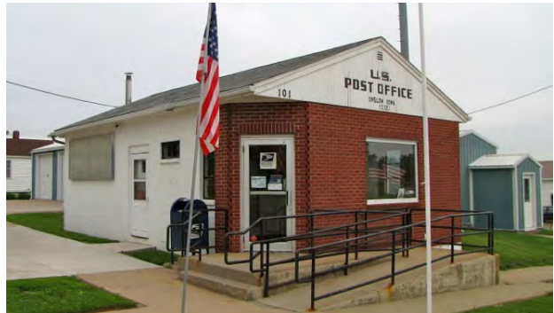
5 GRADE CONCRETE BLOCK – WOOD FRAME
