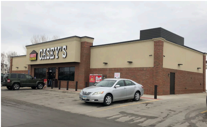
2 GRADE BRICK VENEER – WOOD FRAME
