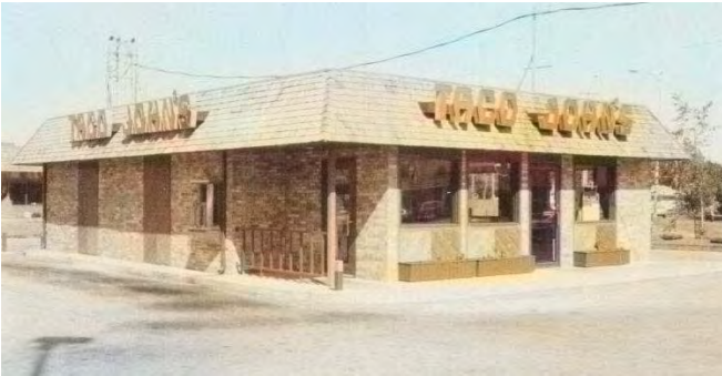
3 GRADE BRICK VENEER – WOOD FRAME
