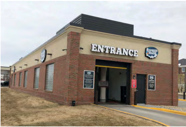
2 GRADE – DRIVE THRU BRICK – STEEL FRAME
