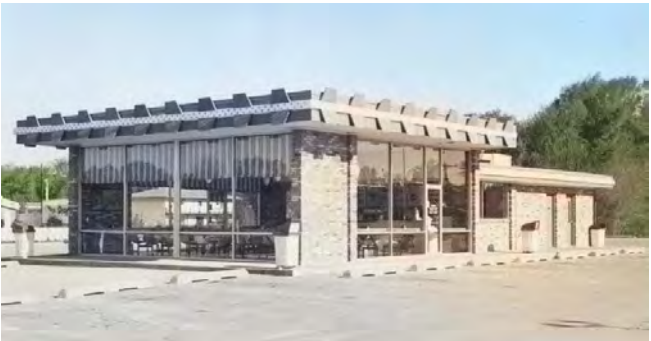
4 GRADE BRICK VENEER – STEEL FRAME
