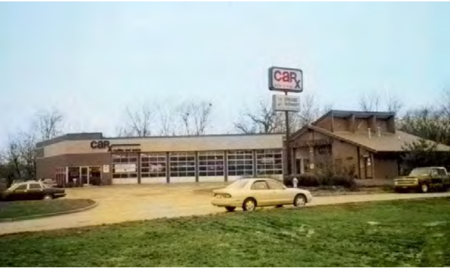
3 GRADE BRICK ON BLOCK – STEEL FRAME
