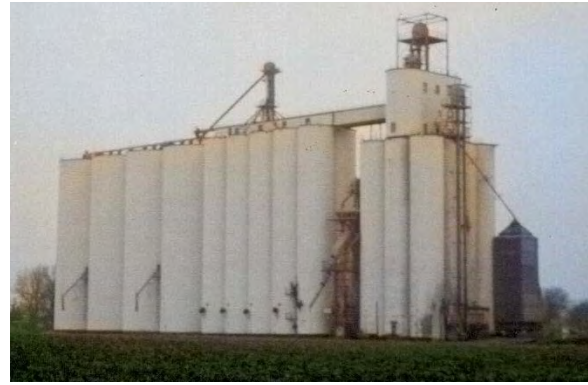
CONCRETE ELEVATOR WITH CONCRETE ANNEX
