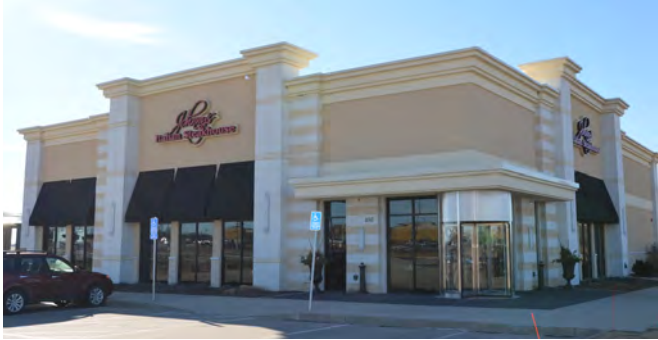
1 GRADE EIFS – WOOD FRAME
