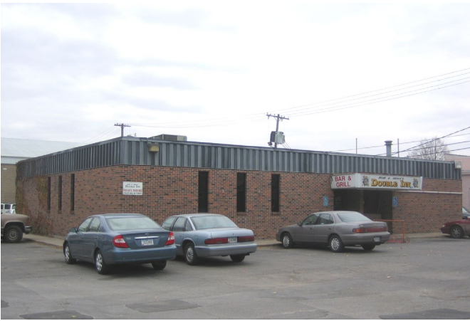
4 GRADE BRICK ON BLOCK – STEEL FRAME
