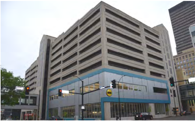
2 GRADE REINFORCED CONC. – REINFORCED CONCRETE FRAME
