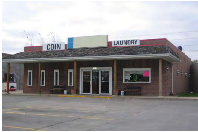
4 GRADE BRICK ON BLOCK – STEEL FRAME
