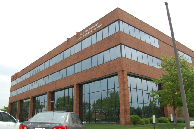
2 GRADE BRICK ON BLOCK – STEEL FRAME
