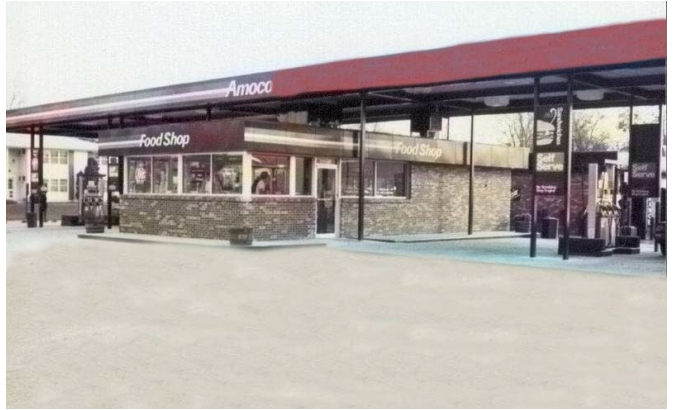
4 GRADE BRICK ON BLOCK – STEEL FRAME
