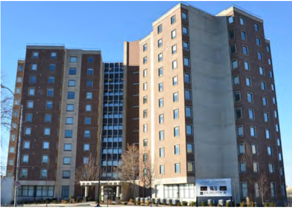
2 GRADE BRICK – CONCRETE FRAME
