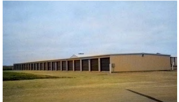
4 GRADE METAL – LIGHT STEEL FRAME
