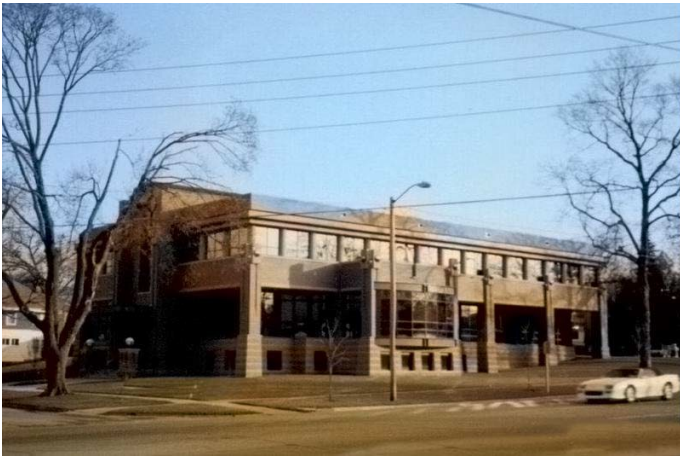
2 + 10 GRADE BRICK – STEEL FRAME
