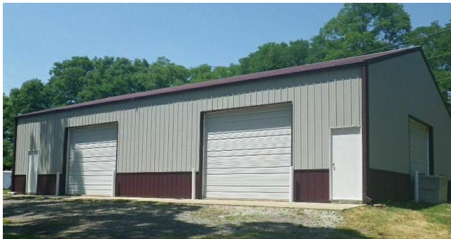
4 GRADE METAL WAREHOUSE – POST FRAME
