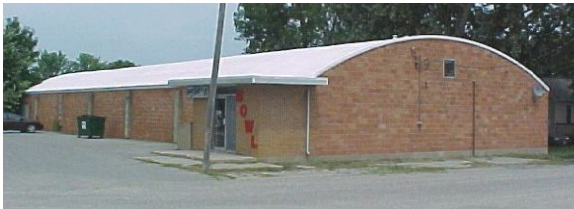
5 GRADE TILE (CONCRETE BLOCK) – WOOD FRAME
