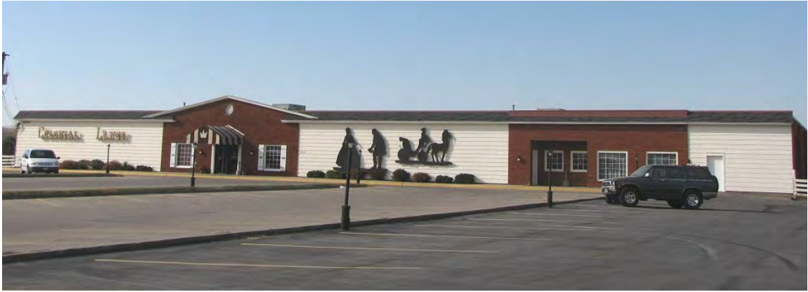
4 + 10 GRADE CONCRETE BLOCK – STEEL FRAME
