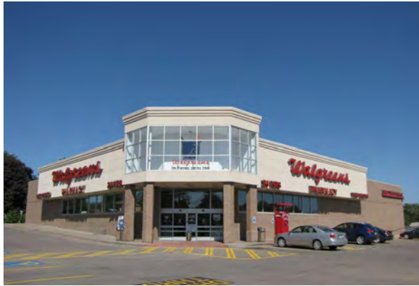
3 GRADE BRICK ON BLOCK – STEEL FRAME
