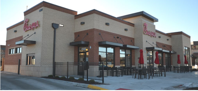
1 GRADE BRICK VENEER – WOOD FRAME
