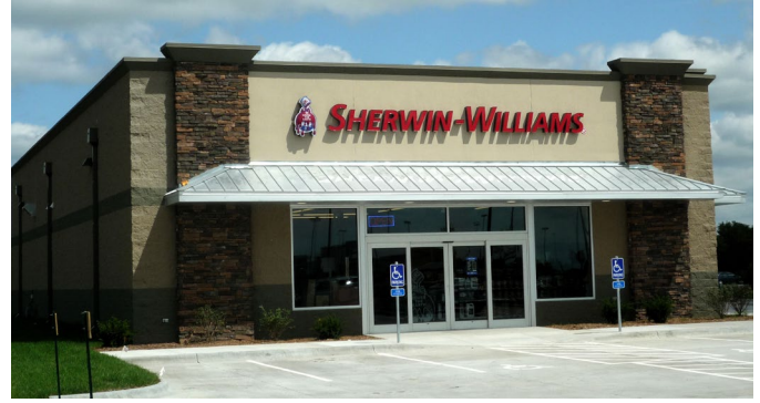
2 GRADE DECORATIVE CONCRETE BLOCK – STEEL FRAME
