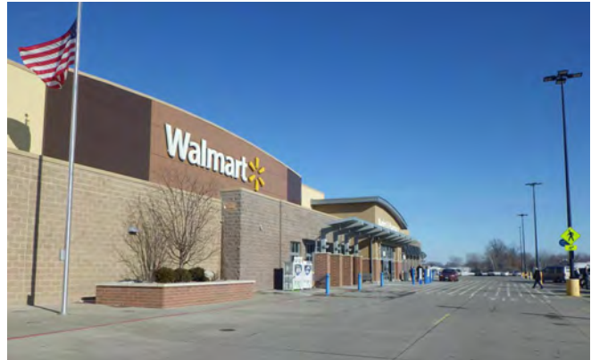
3 GRADE CONCRETE TILT-UP – STEEL FRAME
