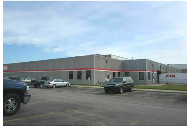
4 + 10 GRADE CONCRETE TILT-UP – STEEL FRAME
