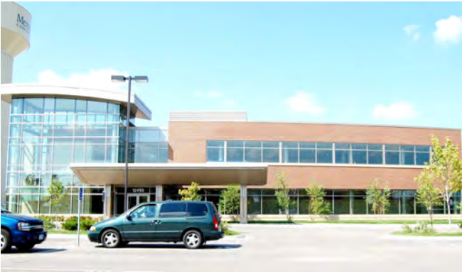
1 GRADE BRICK VENEER – STEEL FRAME
