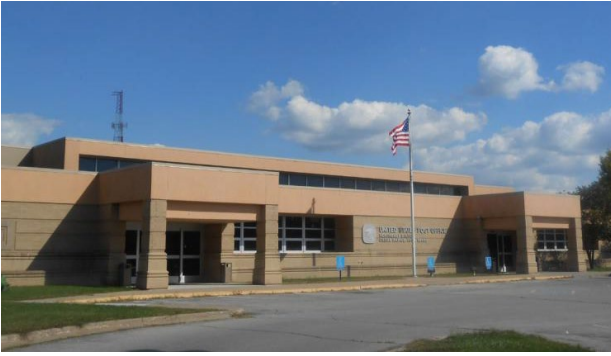
2 GRADE BRICK ON BLOCK – STEEL FRAME
