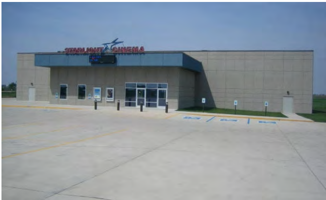
4 GRADE CONCRETE TILT-UP – STEEL FRAME
