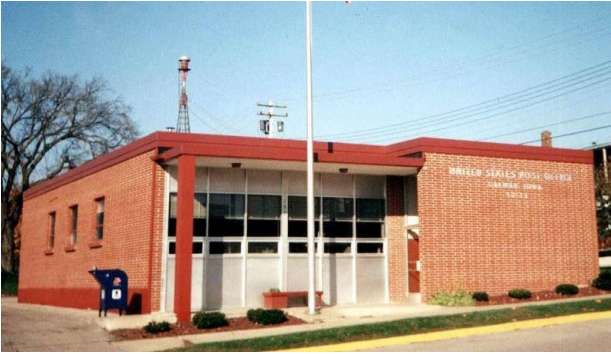
4 GRADE BRICK ON BLOCK – STEEL FRAME
