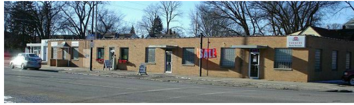
5 GRADE BRICK ON BLOCK – WOOD FRAME
