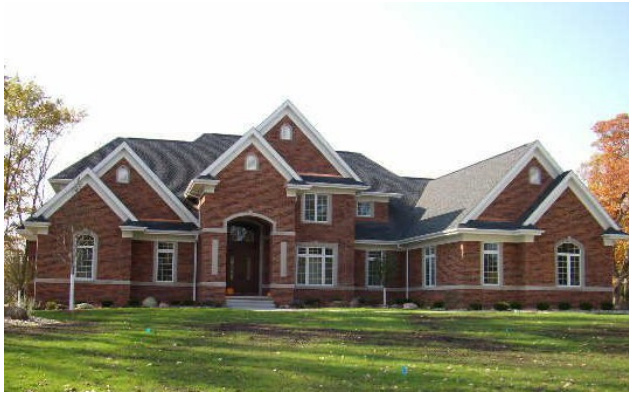
1 + 10 2 STORY + BASEMENT BRICK DWELLING
