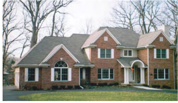
2 + 10 2 STORY + BASEMENT FRAME & BRICK DWELLING
