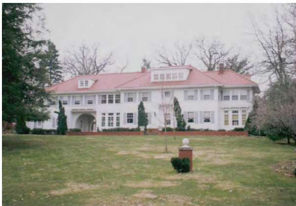
E 2 STORY + ATTIC + BASEMENT BRICK DWELLING
