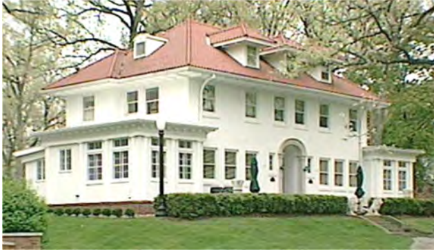
1 2 STORY + ATTIC + BASEMENT BRICK DWELLING
