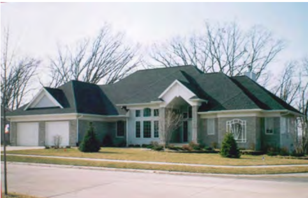
2 + 5 1 STORY + BASEMENT FRAME & BRICK DWELLING
