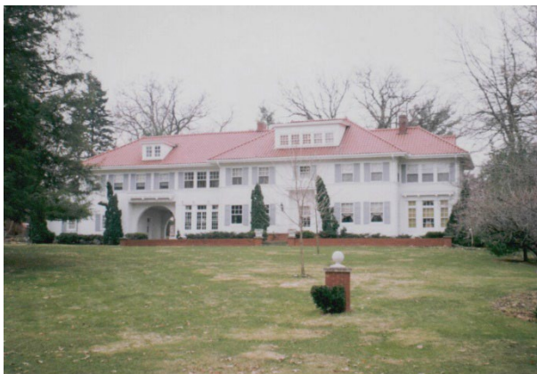
E 2 STORY + ATTIC + BASEMENT BRICK DWELLING
