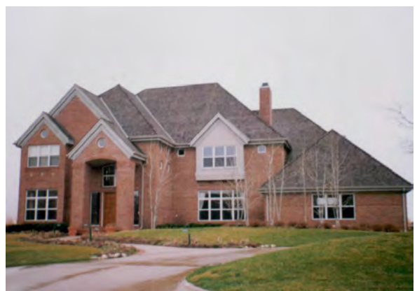
1 2 STORY + BASEMENT BRICK DWELLING
