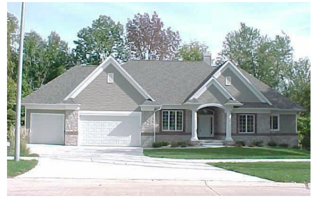
2 + 5 1 STORY + BASEMENT FRAME & BRICK DWELLING
