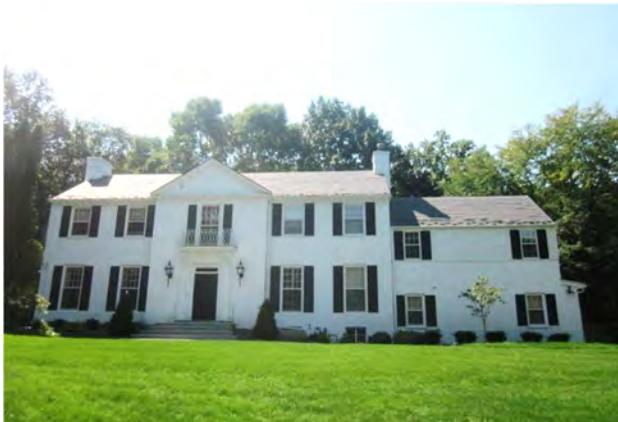
1 - 10 2 STORY + BASEMENT BRICK DWELLING
