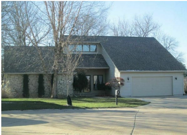
3 + 10 1 ½ STORY + BASEMENT FRAME DWELLING
