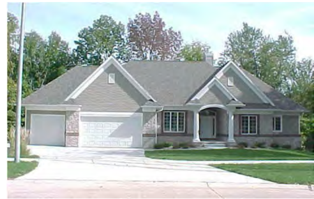
2 + 5 1 STORY + BASEMENT FRAME & BRICK DWELLING
