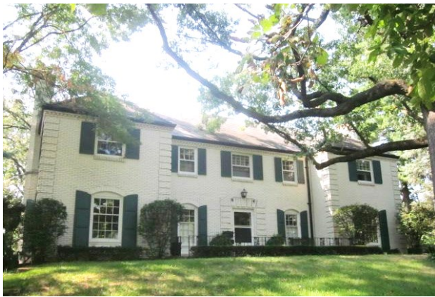
1 - 5 2 STORY + BASEMENT BRICK DWELLING
