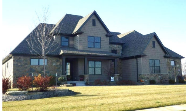
1 - 5 2 STORY + BASEMENT FRAME AND STONE DWELLING
