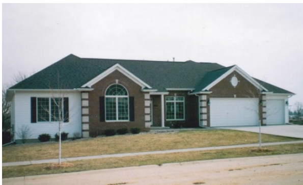
2 - 10 1 STORY + BASEMENT FRAME & BRICK DWELLING
