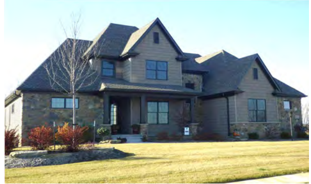
1 - 5 2 STORY + BASEMENT FRAME AND STONE DWELLING
