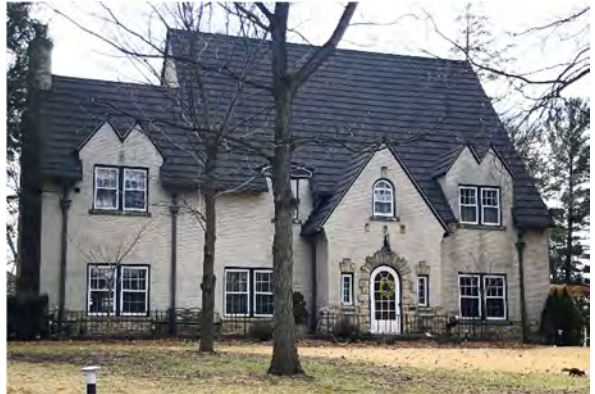
1 + 10 2 STORY + BASEMENT BRICK DWELLING
