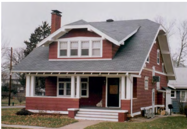
4 + 10 1 ½ STORY + BASEMENT FRAME DWELLING
