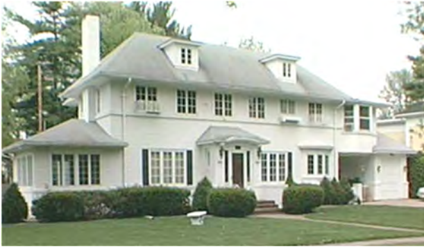
2 + 10 2 STORY + ATTIC + BASEMENT BRICK DWELLING
