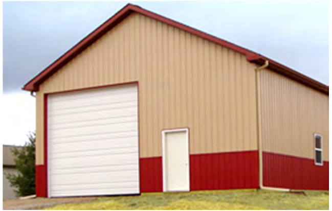
4 GRADE METAL POST FRAME HIGH BAY GARAGE
