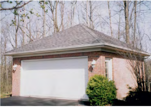
3 GRADE BRICK GARAGE
