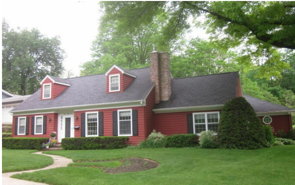
3 1 ½ STORY + BASEMENT FRAME DWELLING
