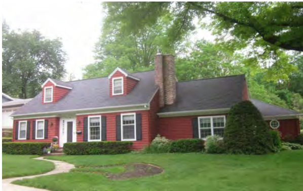
3 1 ½ STORY + BASEMENT FRAME DWELLING
