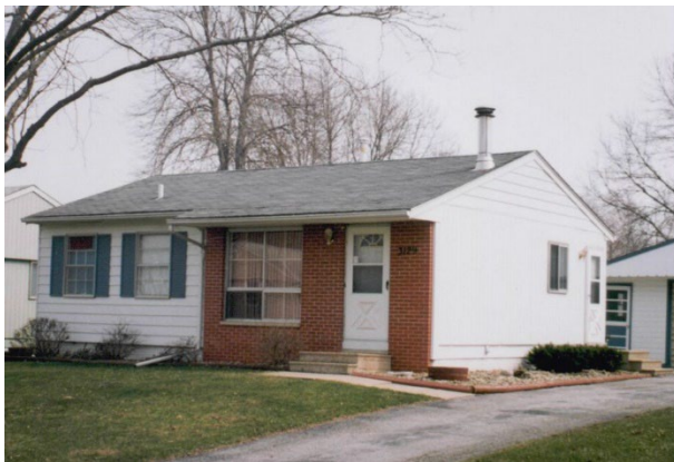
4 - 10 1 STORY + BASEMENT FRAME & BRICK DWELLING
