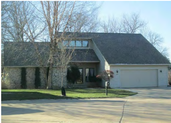
3 + 10 1 ½ STORY + BASEMENT FRAME DWELLING
