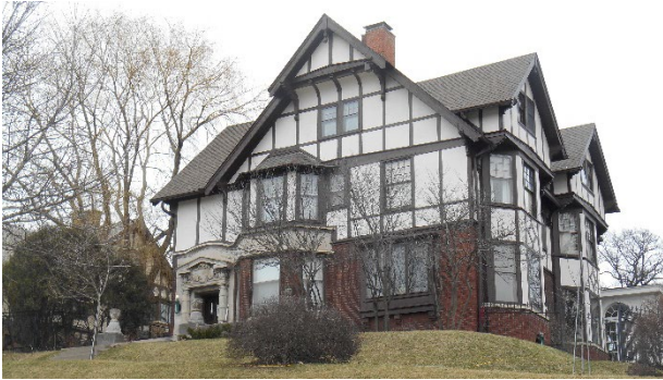
2 + 10 2 ½ STORY + BASEMENT FRAME & BRICK DWELLING
