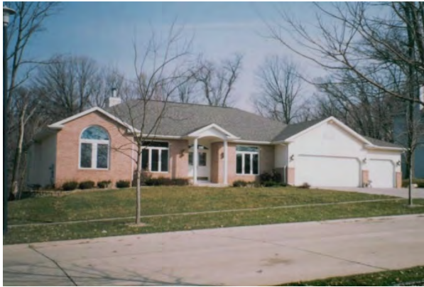
2 - 5 1 STORY + BASEMENT FRAME & BRICK DWELLING
