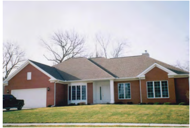
2 1 STORY + BASEMENT FRAME & BRICK DWELLING
