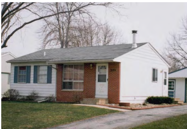
4 - 10 1 STORY + BASEMENT FRAME & BRICK DWELLING
