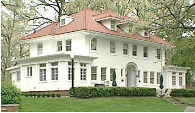
1 2 STORY + ATTIC + BASEMENT BRICK DWELLING
