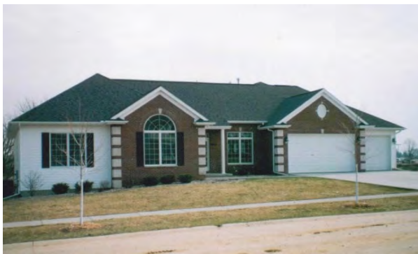
2 - 10 1 STORY + BASEMENT FRAME & BRICK DWELLING
