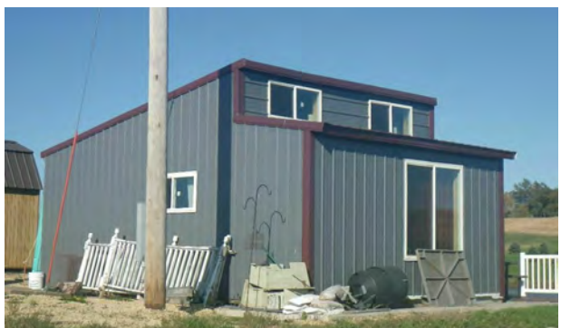
6 1 STORY METAL POST FRAME DWELLING (LOW QUALITY INTERIOR)
