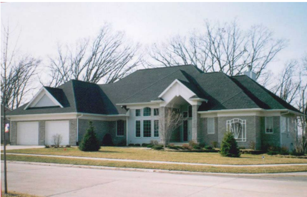
2 + 5 1 STORY + BASEMENT FRAME & BRICK DWELLING
