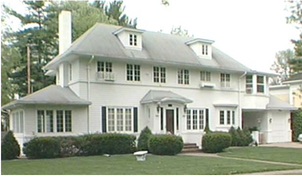
2 + 10 2 STORY + ATTIC + BASEMENT BRICK DWELLING
