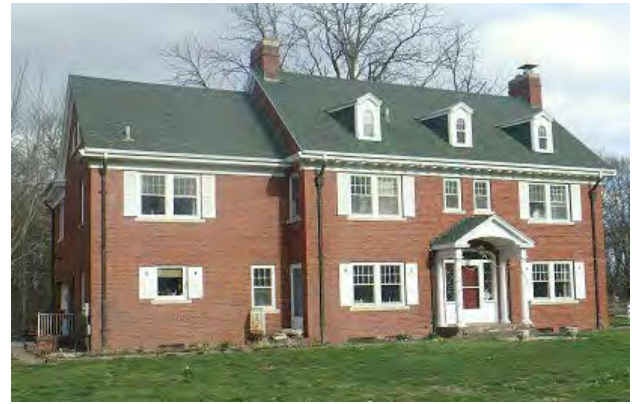
2 - 5 2 STORY + BASEMENT BRICK DWELLING
