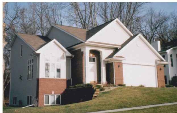
3 - 5 1 ½ STORY + BASEMENT FRAME AND BRICK DWELLING
