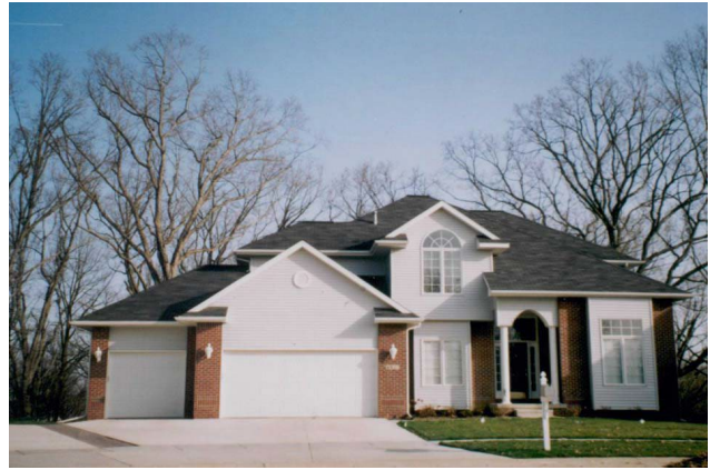
3 + 10 2 STORY + BASEMENT FRAME & BRICK DWELLING
