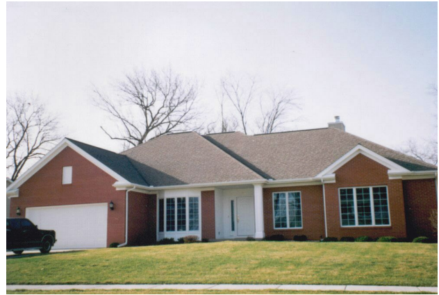
2 1 STORY + BASEMENT FRAME & BRICK DWELLING
