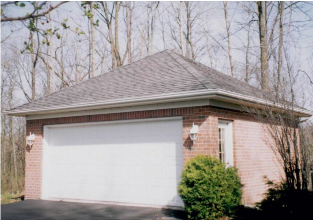
3 GRADE BRICK GARAGE
