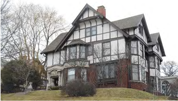
2 + 10 2 ½ STORY + BASEMENT FRAME & BRICK DWELLING
