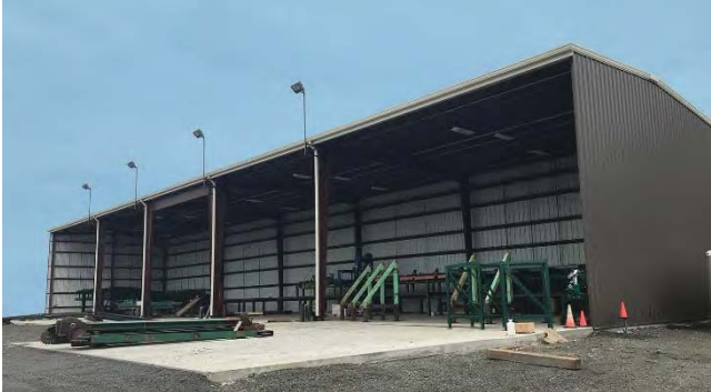
4 GRADE RIGID STEEL FRAME (OPEN SIDEWALL)
