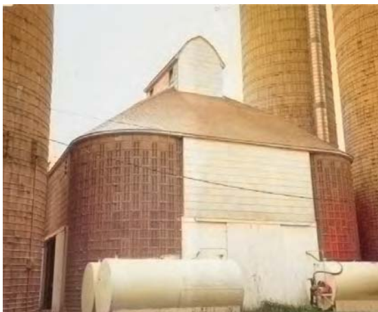
3+10 GRADE CONCRETE STAVE DOUBLE CRIB
