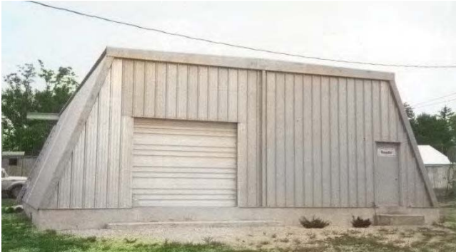
4 GRADE STEEL FRAME SLANT WALL
