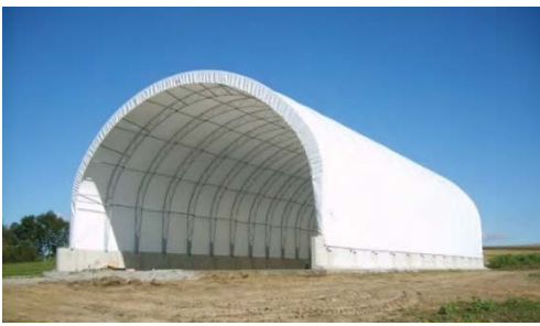
HOOP HOUSE W/ CONCRETE PONY WALL
