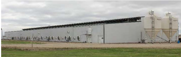
4 GRADE 2 STORY METAL PULLET BUILDING
