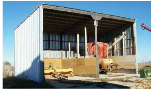
METAL – POST FRAME W/ WOOD DIVIDERS
