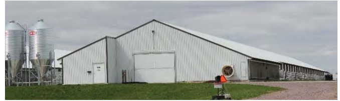
4 GRADE 1 STORY METAL PULLET BUILDING
